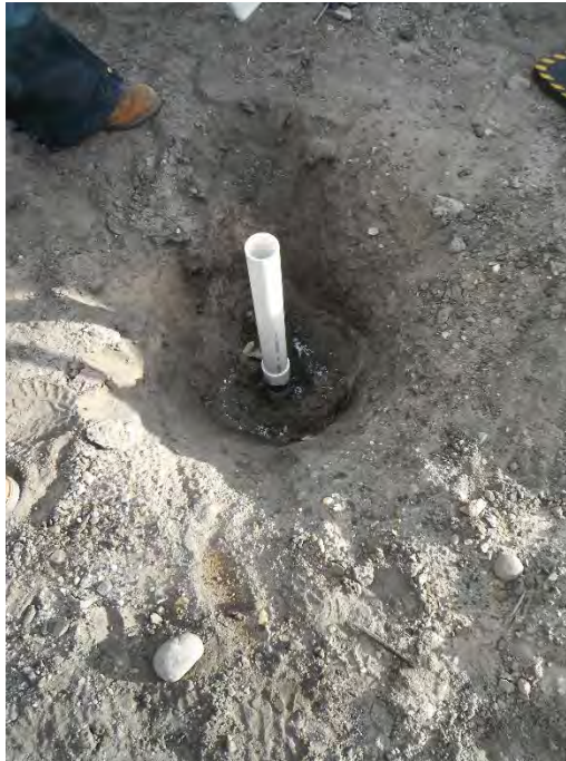
No. 11 – INTERA staff added 3 feet of 2-inch diameter PVC casing to the top of monitoring well MW-02. The top of casing elevation was re-surveyed after the modifications.
