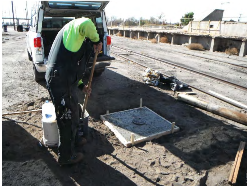
No. 13 – INTERA staff pouring the ground-flush cement apron around monitoring well MW-02.
