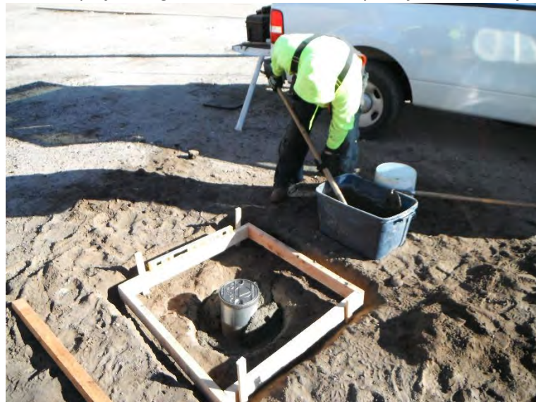
No. 11 – INTERA staff added 3 feet of 2-inch diameter PVC casing to the top of monitoring well MW-02. The top of casing elevation was re-surveyed after the modifications.
