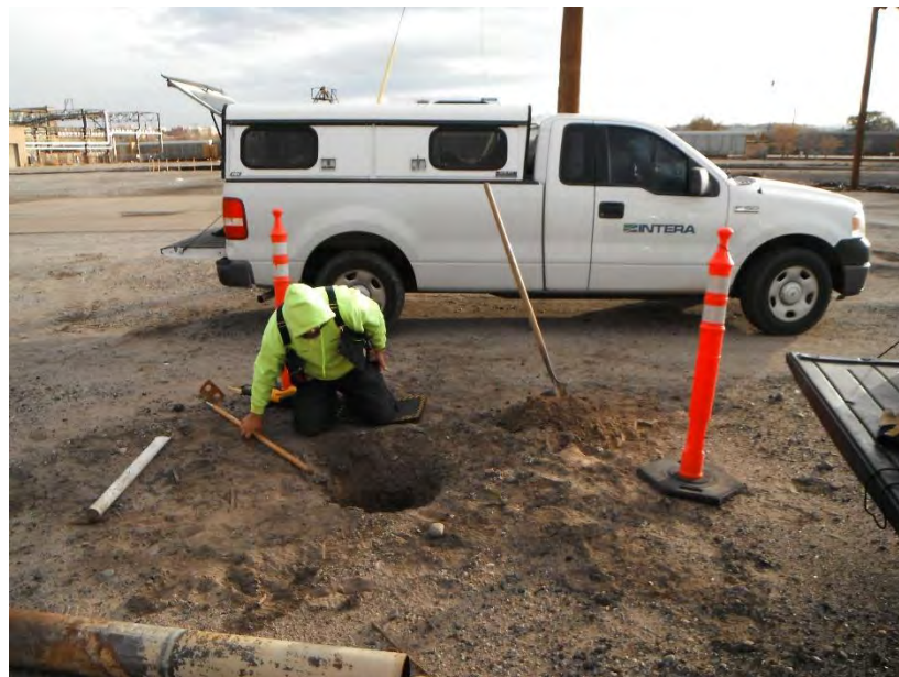
No. 10 – INTERA staff preparing to modify the surface completion at monitoring well MW-02. December 2016.
