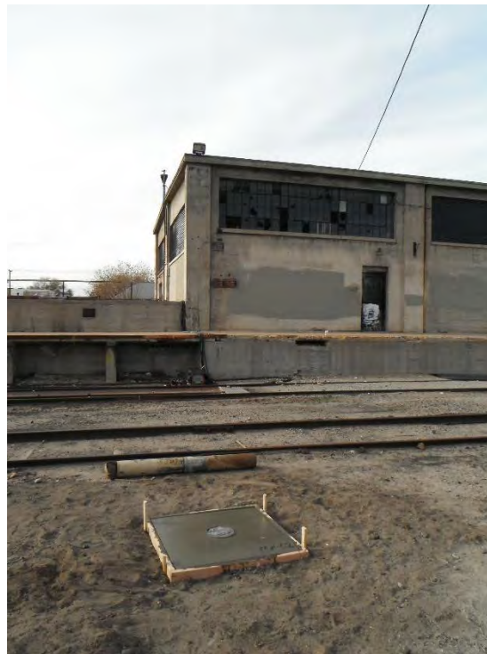
No. 14 – Monitoring well MW-02 surface completion as of December 2016.
