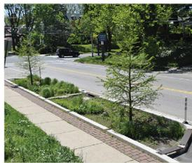
**Stormwater Bumpout:** An area for rain water capture and infiltration created when the curb and gutter is moved out into the portion of the roadway normally reserved for parking. Otherwise known as 'bulbouts', 'chicanes', and 'curb extensions'. Also slows traffic. (credit: Bernillo County GSI LID Standards, 2021)
