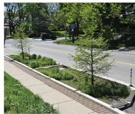
**Stormwater Bumpout:** An area for rain water capture and infiltration created when the curb and gutter is moved out into the portion of the roadway normally reserved for parking. Otherwise known as 'bulbouts', 'chicanes', and 'curb extensions'. Also slows traffic. (credit: Bemalillo County GSI LID Standards, 2021)
