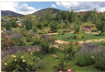
**Stormwater Harvesting Basin:** GSI practice consisting of a shallow vegetated basin designed for capture and infiltration of stormwater runoff to support vegetation and improve water quality. (credit: Bemalillo County GSI LID Standards, 2021)
