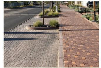
**Permeable Pavement:** Paving material that allows stormwater to move through the pavement's surface to a storage layer below, allowing infiltration into the underlying soil. Material options include porous asphalt, pervious concrete, pavers, and various plastic products for reinforcing gravel or grass. (credit: Bemalillo County GSI LID Standards, 2021)
