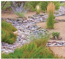
**Bio Swale:** GSI practice consisting of a shallow, linear feature designed to improve water quality by conveying, slowing, and treating runoff; allows pollutants to settle out and promotes infiltration. (credit: Bemalillo County GSI LID Standards, 2021)
