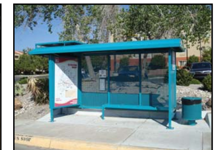
Enhanced bus stops with branded/themed shelters, ADA compliant platforms, lighting and route info help emphasize South Yale Boulevard as a key transit corridor
