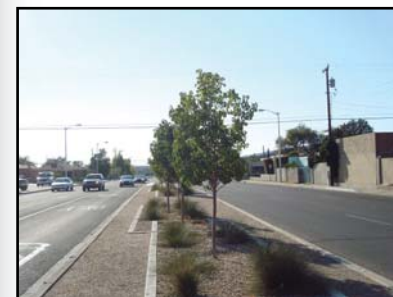
Raised medians provide area for water-conservative, native landscaping and can provide traffic calming and aesthetic benefits, as well as space to locate pedestrian safety measures and amenities.
