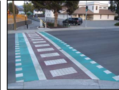
Alternative paving or imprinting materials can be used at crosswalks and within intersections to increase visibility and identify a unique area
