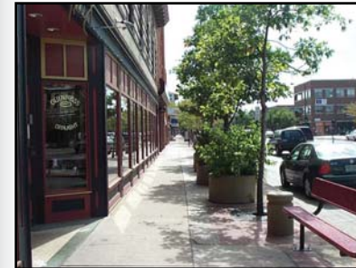
Widened sidewalk provide additional width for pedestrian movement and expand the pedestrian realm to include trees, street furniture, and other amenities
