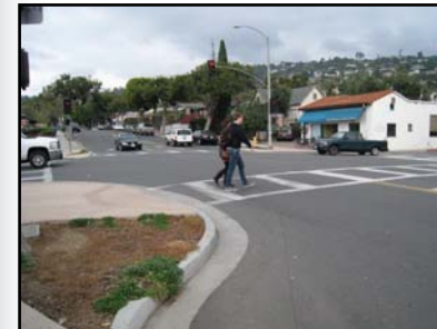
Curb extensions ("bulbouts") shorten crossing distances for pedestrians and provide area for landscaping, benches, street art, etc.
