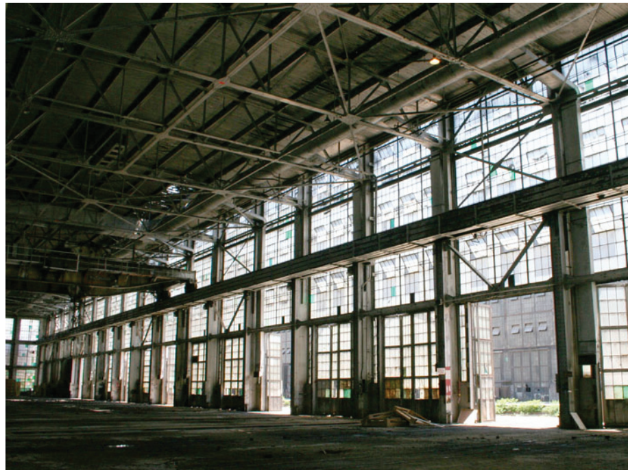
Boiler Shop, Bay #1, Fully Glazed southern elevation with 18' tall operable doors.
