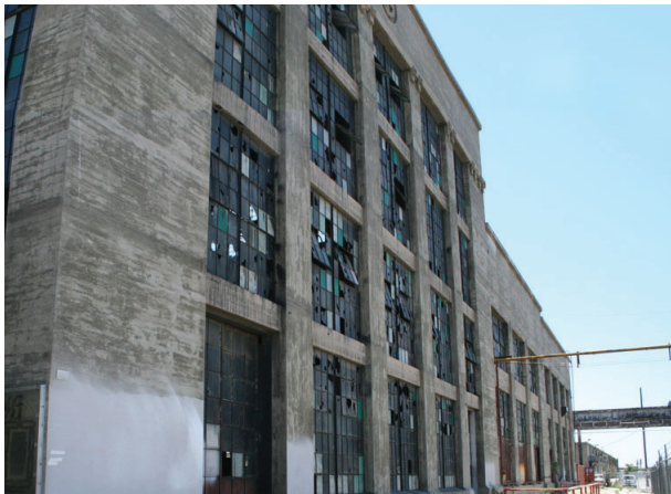
West Elevation, Cast in Place Concrete Frame.
