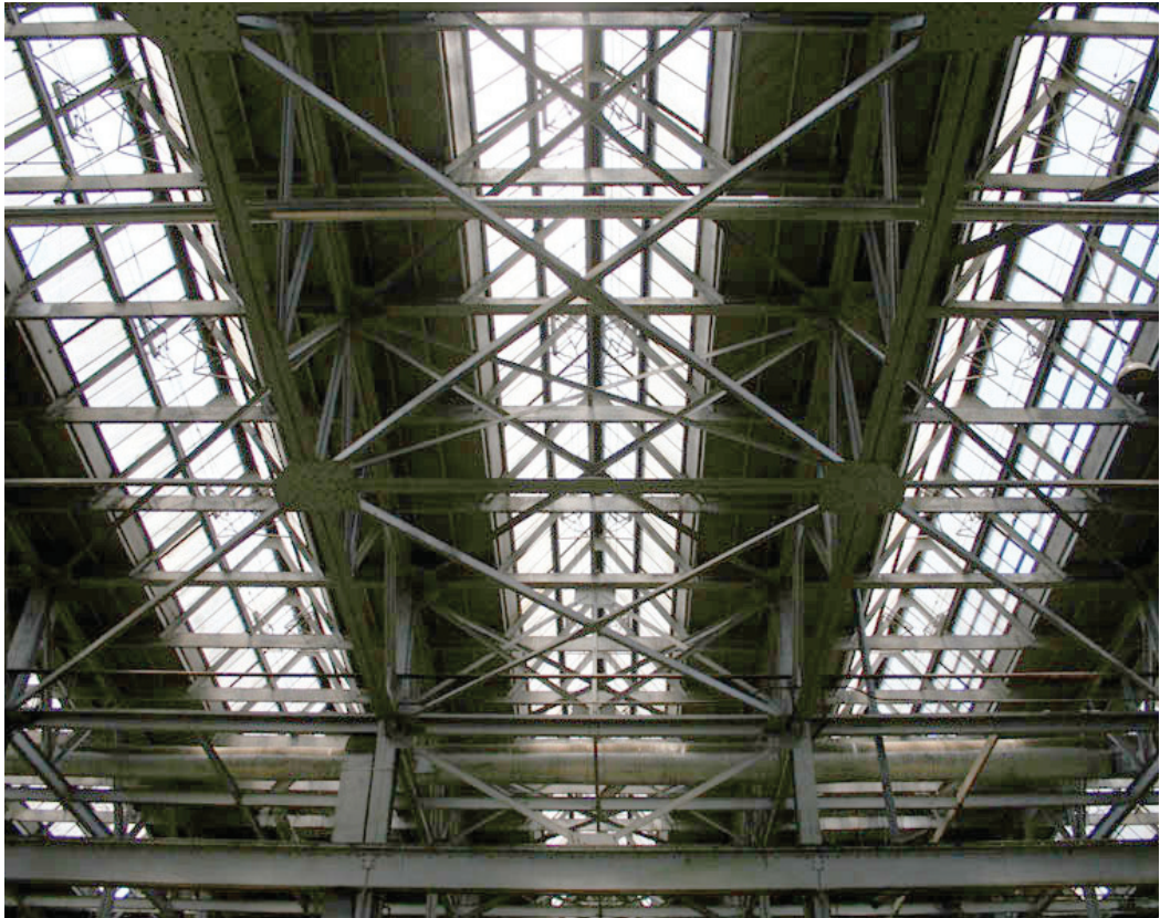
Machine Shop, Pyramidal skylights over Bays 2 and 3.
