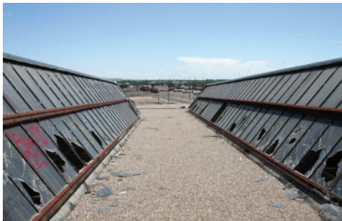
Built-up roofing, positive slope to South.
