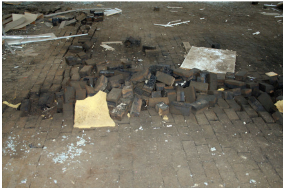
Damaged flooring, 3" thick creosoted end-grain wood blocks
