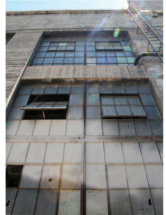
West elevation, Glazing inset to concrete frame.
