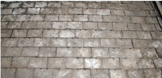
Flooring, 3" thick creosoted end-grain wood blocks.
