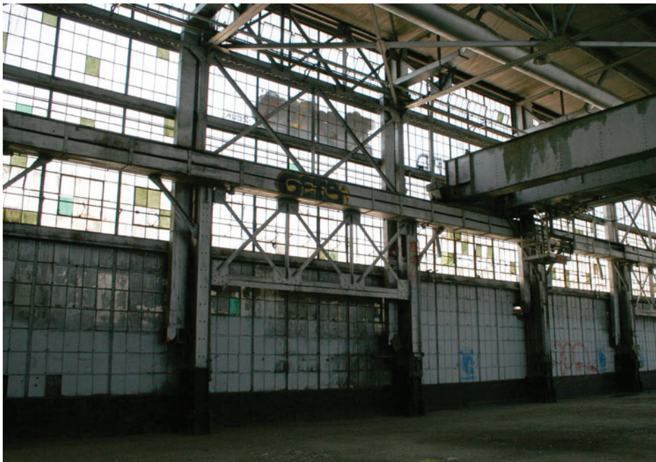
Interior view, West fully glazed elevation with lower 15' blocked by non-original adjacent building.
