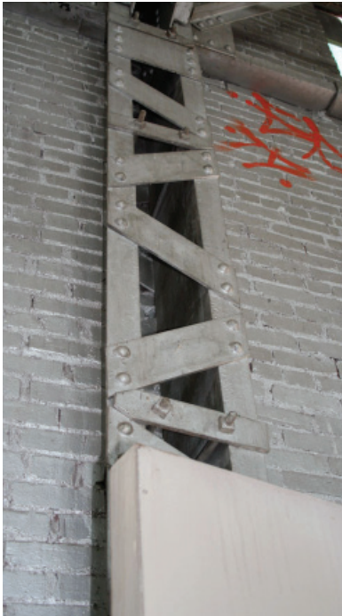
Steel 'trussed' column.
