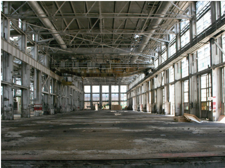
Boiler Shop, Bay #1, Fully Glazed southern elevation, Crane at rear. Floor troughs seen across floor.
