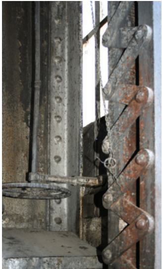
Crank mechanism for skylight operation.
