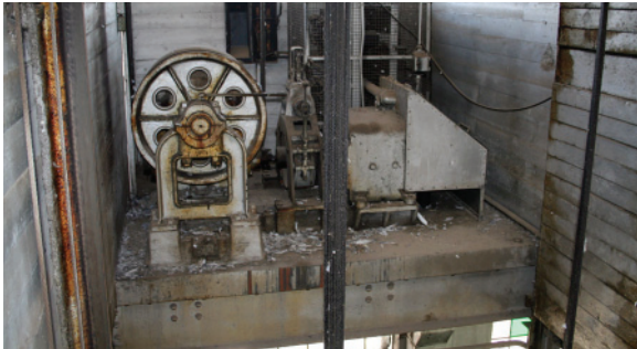
Mezzanine elevator machine room (cab has been removed).
