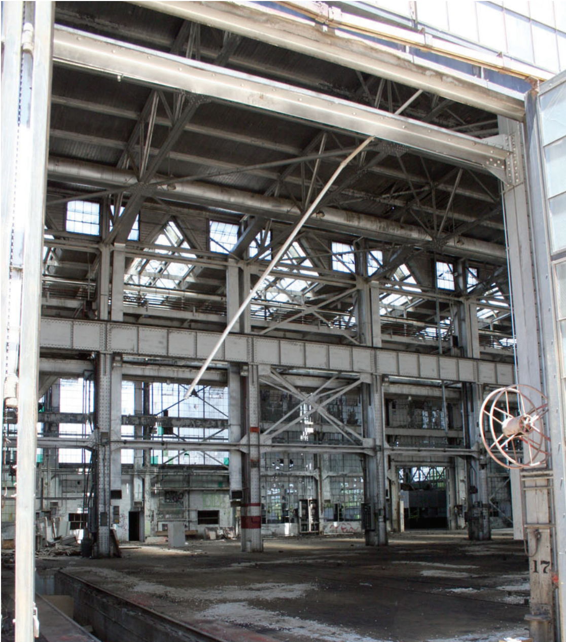
Boiler Shop, View from South Operable Doors
