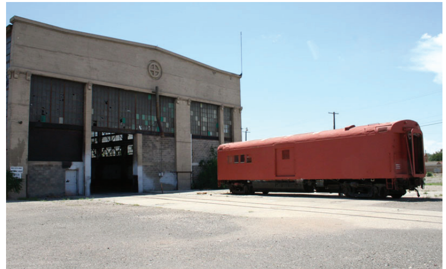
Tank Shop, North elevation.
