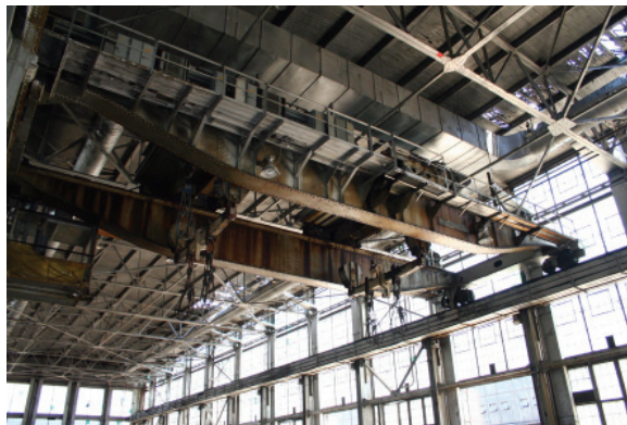
Boiler Shop, Cranes at Bay #1.
