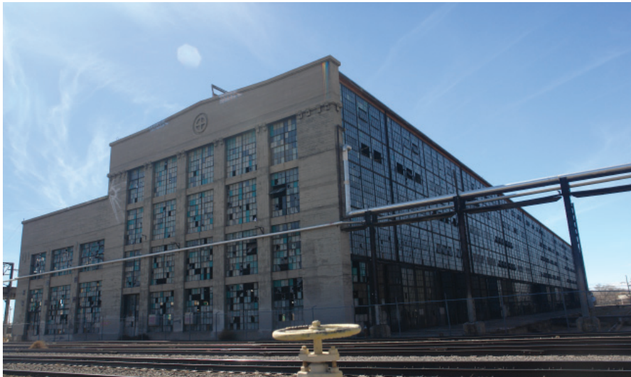
Machine Shop, View Towards West Elevation
