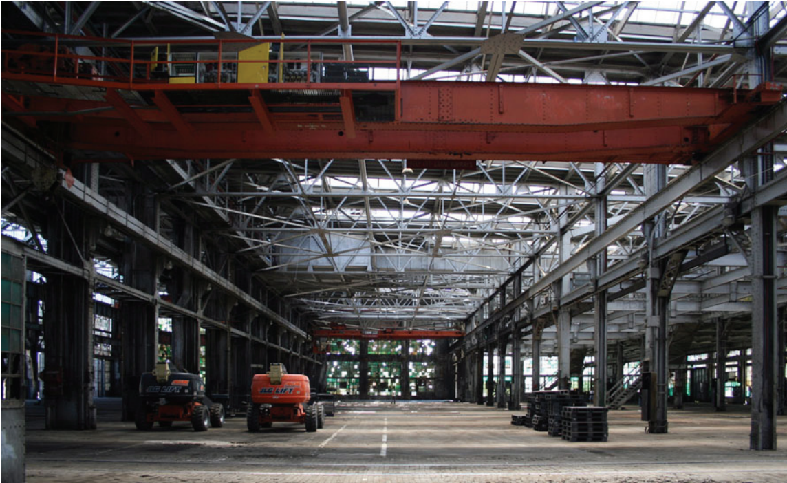
Machine Shop, Bay #3.
