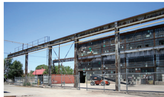
Crane structure extends to 2nd Street.
