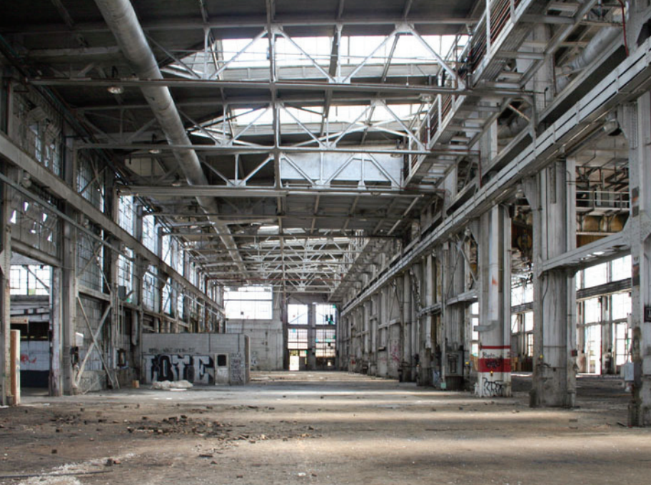
Boiler Shop, Bay #2, Pyramidal skylights
