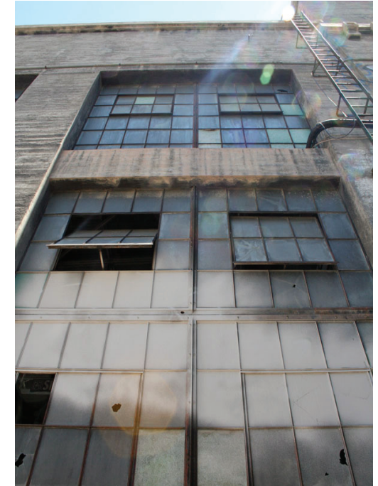
West elevation, Glazing inset to concrete frame.
