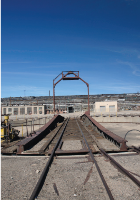
Turntable, View from South.
