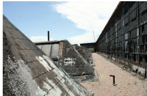
Clerestory skylight at Bay #4.
