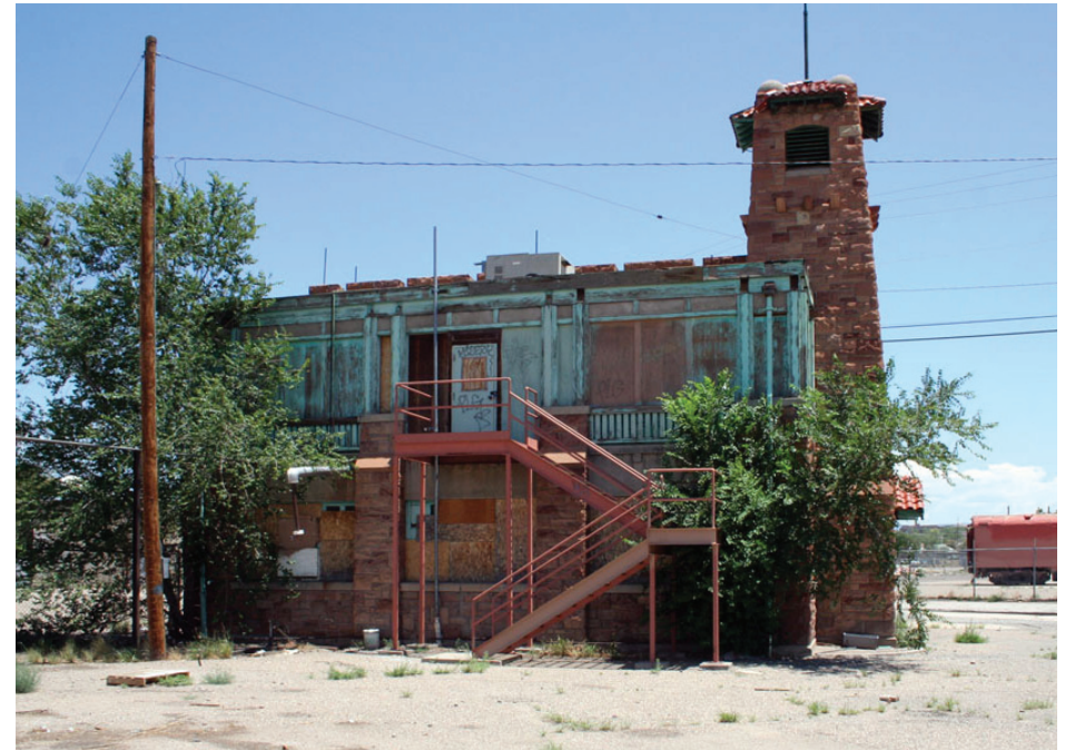
Firehouse, West Elevation.
