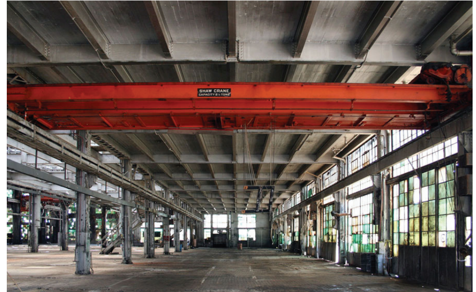
Machine Shop, Bay #1 - Below board formed, cast in place, concrete mezzanine.
