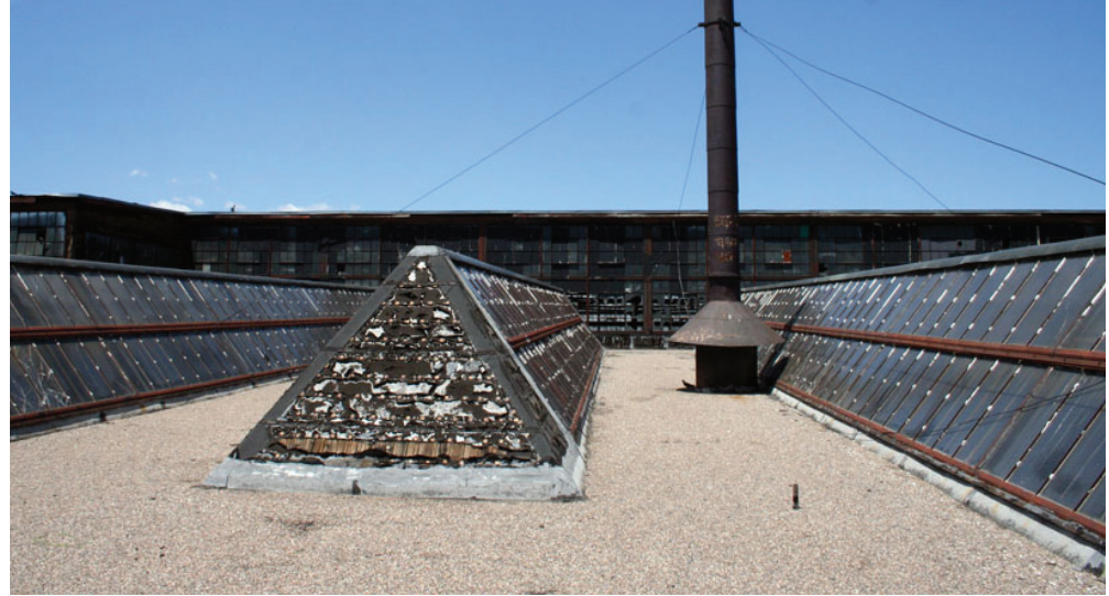
Machine Shop, View from Room looking North.
