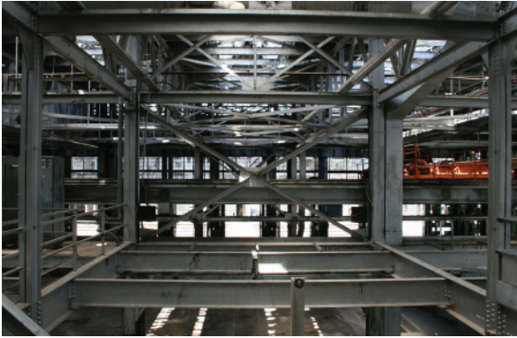
Transverse view from mezzanine.
