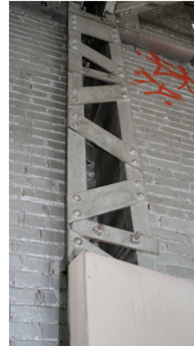
Steel 'trussed' column.
