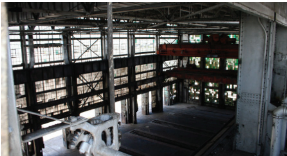
View of Bay #4 from roof clerestory.
