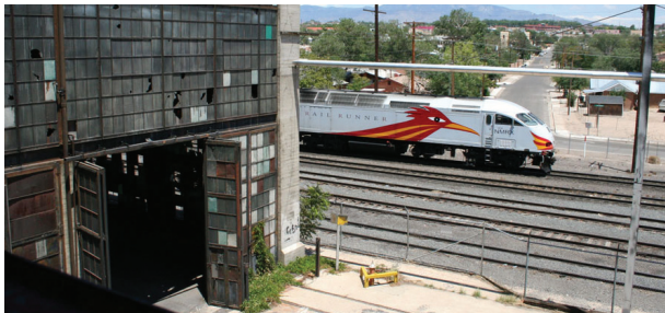
Southeast corner, adjacent active BNSF rail lines .
