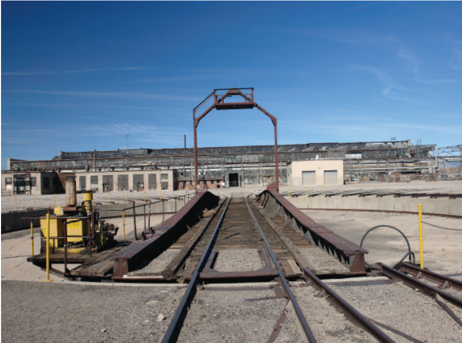
Turntable, View from South.
