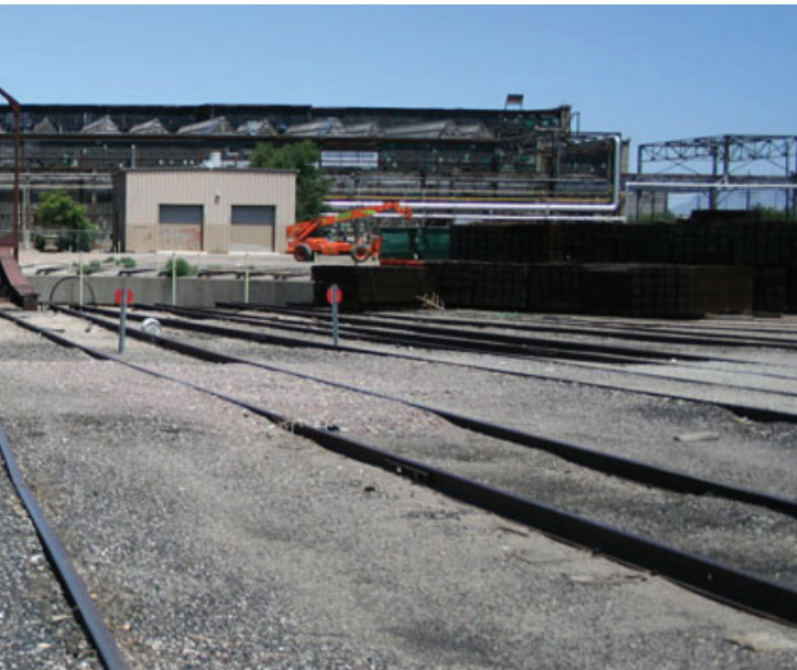
Machine Shop, South Elevation, View across turntable.
