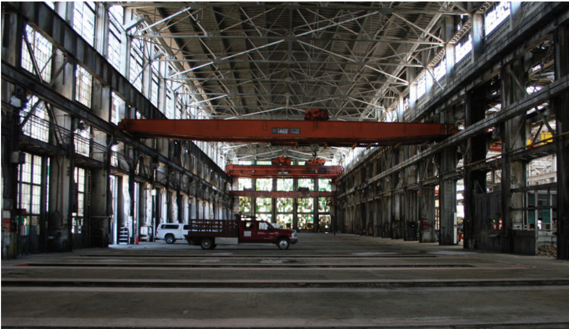
Machine Shop, Bay #4, 57' clear height to underside of truss structure. Floor troughs can be seen across slab.
