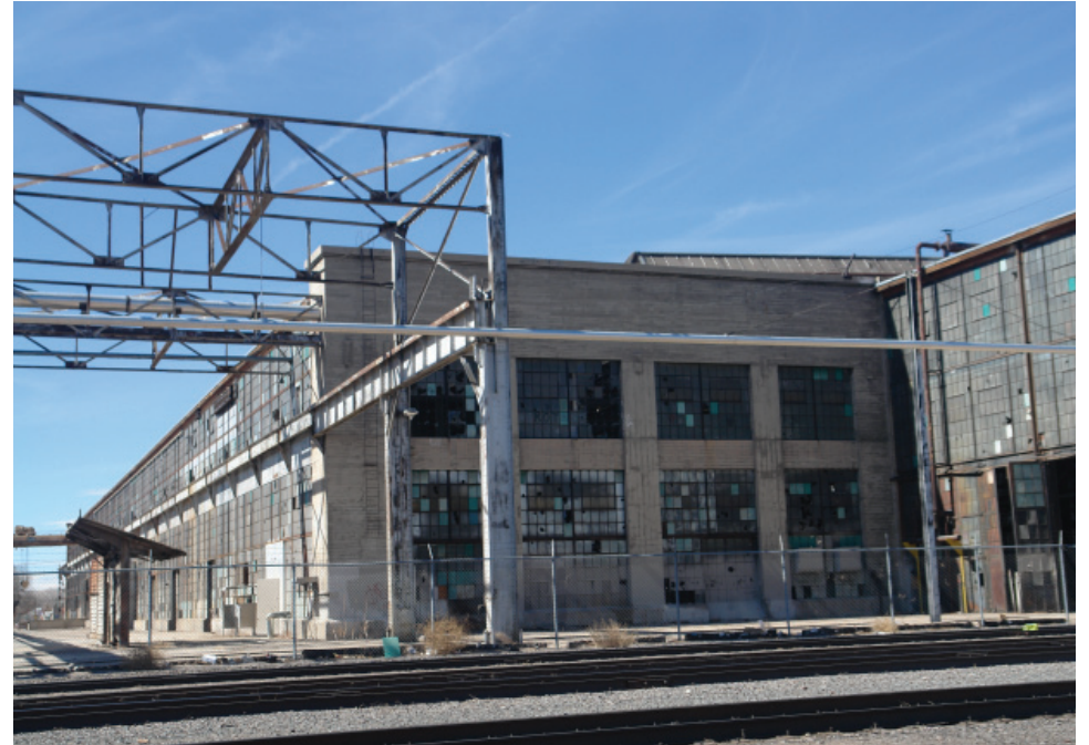
Bridge Crane, View from East Elevation.
