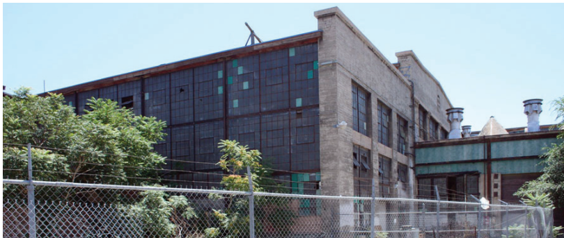
Northeast corner, Reinforced concrete @ fully glazed perimeter wall.
