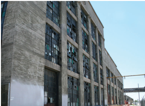
West Elevation, Cast in Place Concrete Frame.
