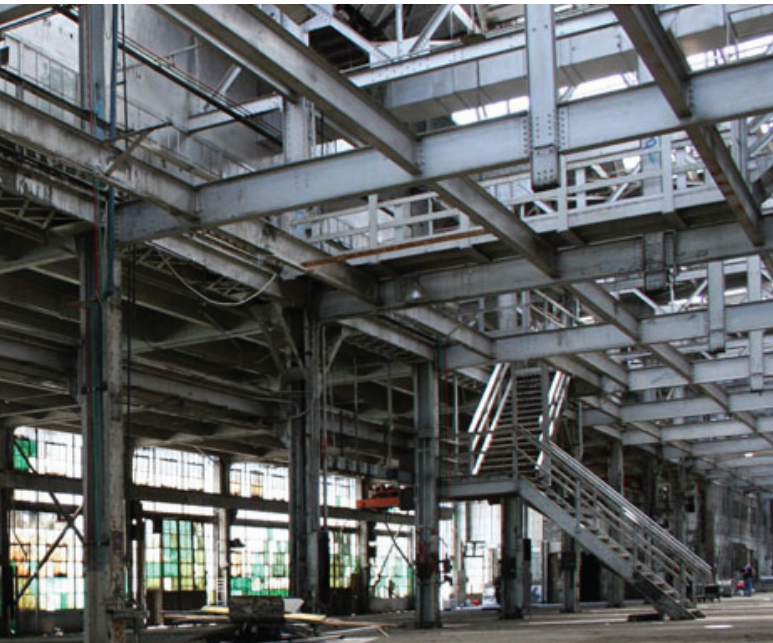
Machine Shop, View up toward mezzanine level.
