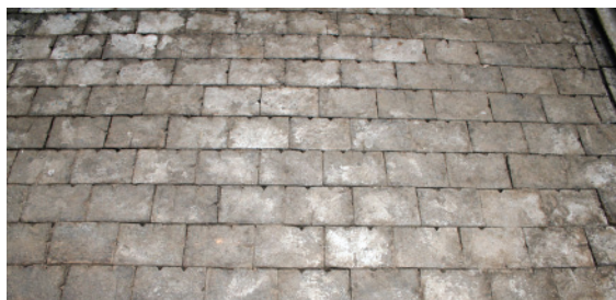
Flooring, 3" thick creosoted end-grain wood blocks.
