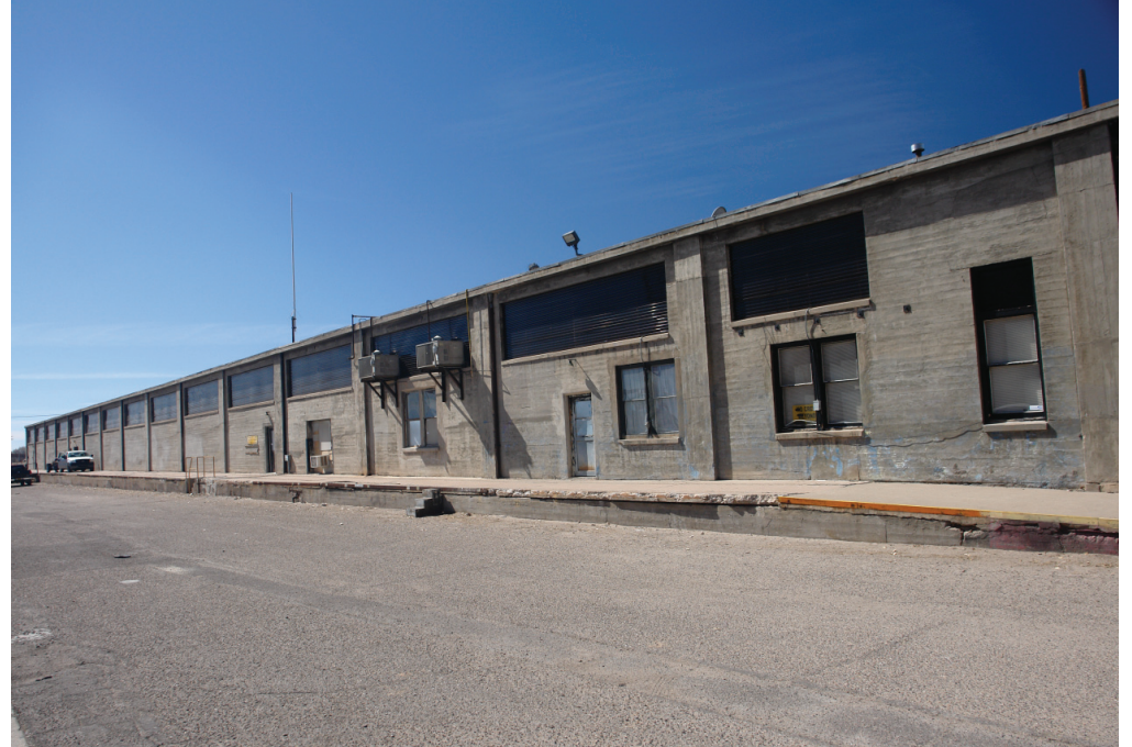
Storehouse, View from North.
