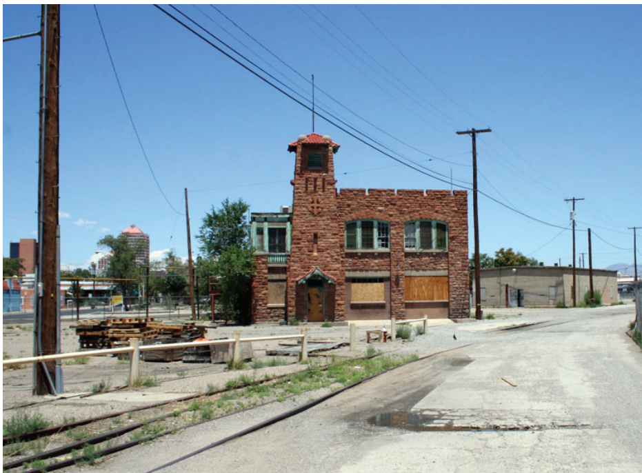
Firehouse, South Elevation.
