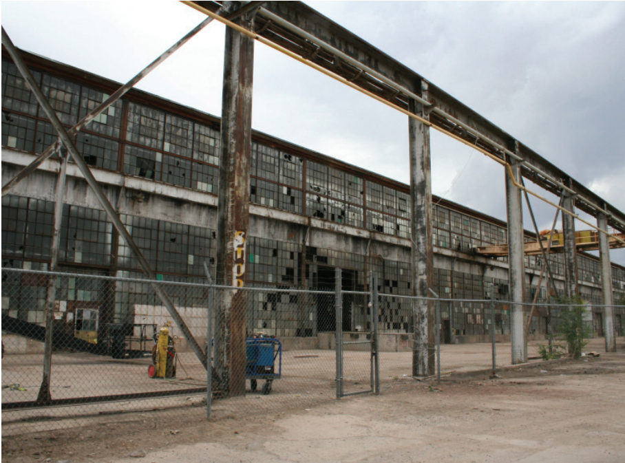
Bridge Crane, View from South West Corner.
