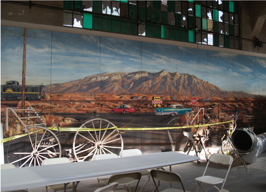
Storehouse, View from Inside.
