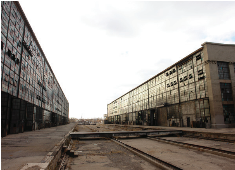
Transfer Table, View from East side.
