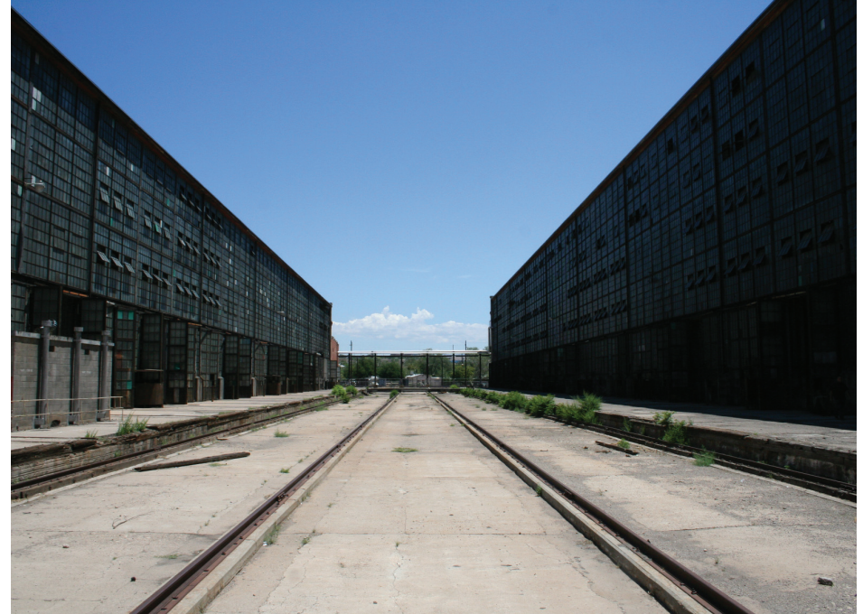
Transfer Table, View from West.
