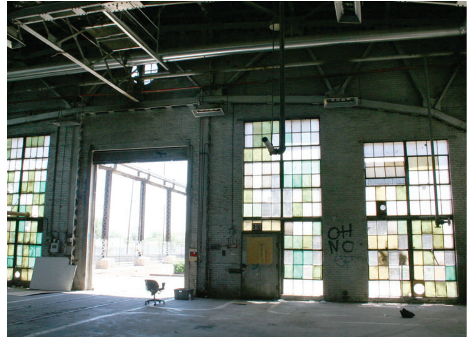
Interior View toward South Elevation Masonry wall.
