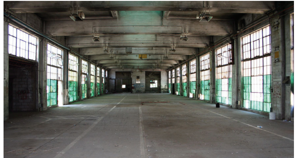
Flue Shop, View down center of Bay.
