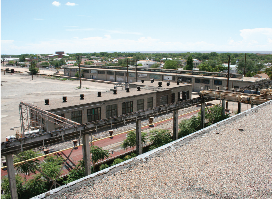
Storehouse, View from roof of Machine Shop.
