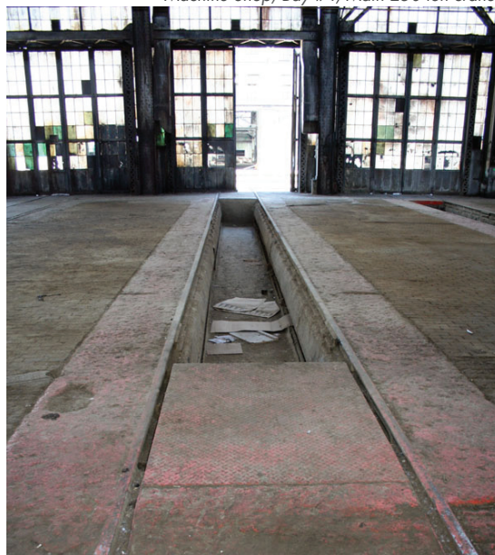
Bay #4, Floor trough.
