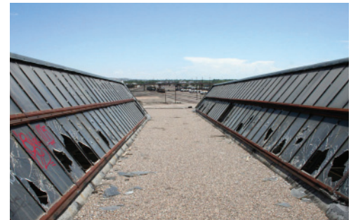
Built-up roofing, positive slope to South.
