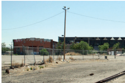
North Elevation from adjacent parcel.
