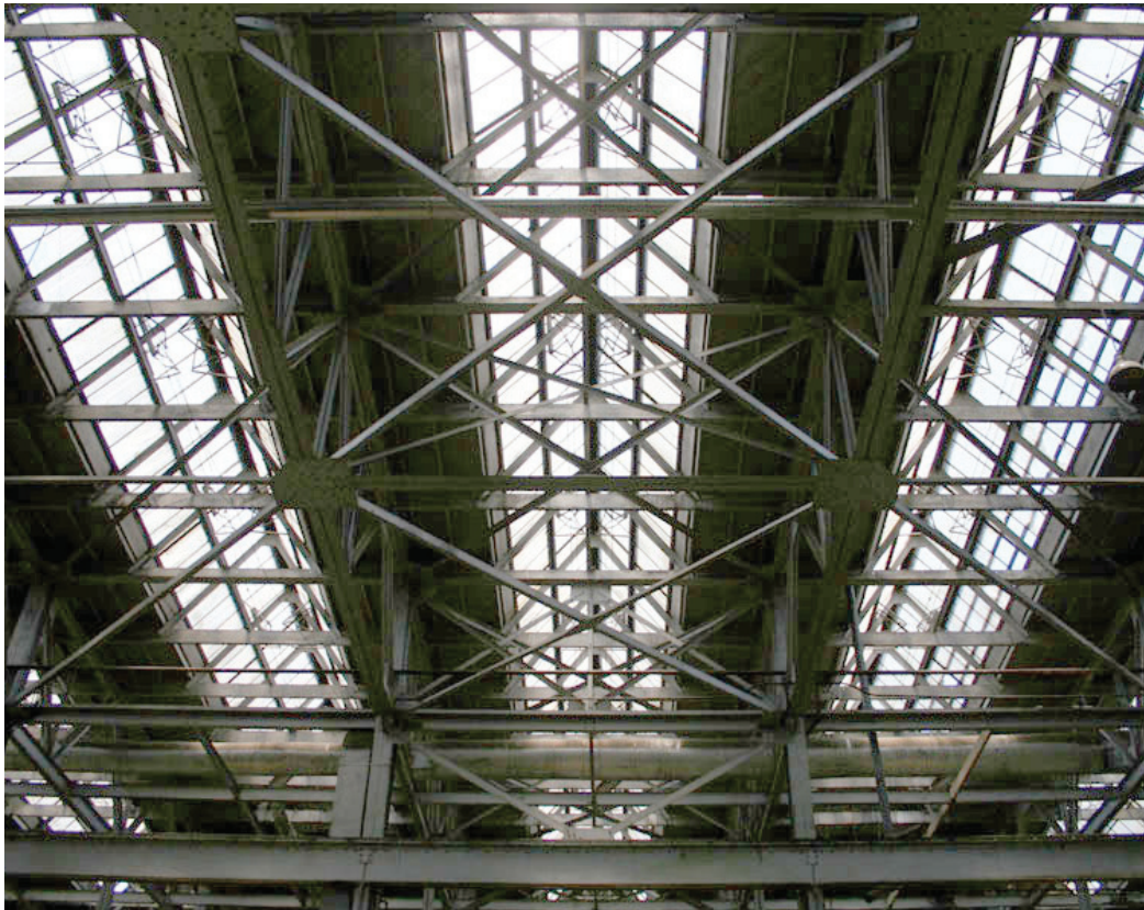
Machine Shop, Pyramidal skylights over Bays 2 and 3.
