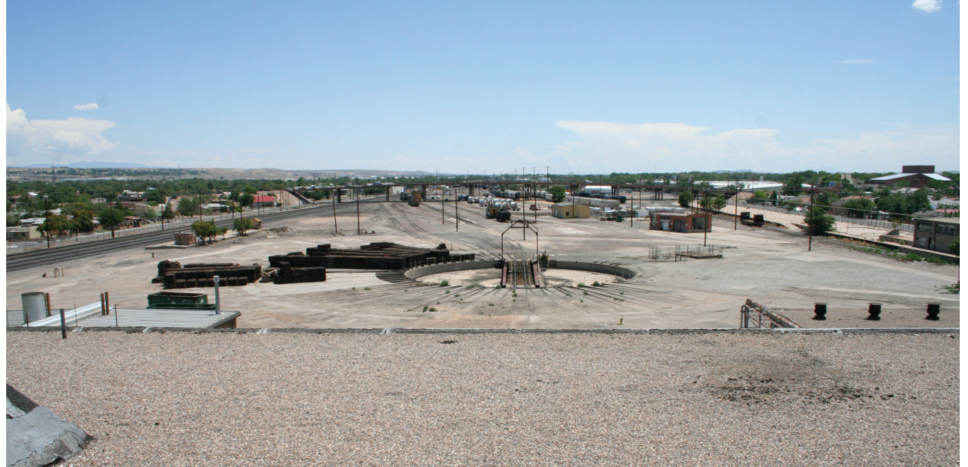
Turntable, View from Machine Shop Roof.
