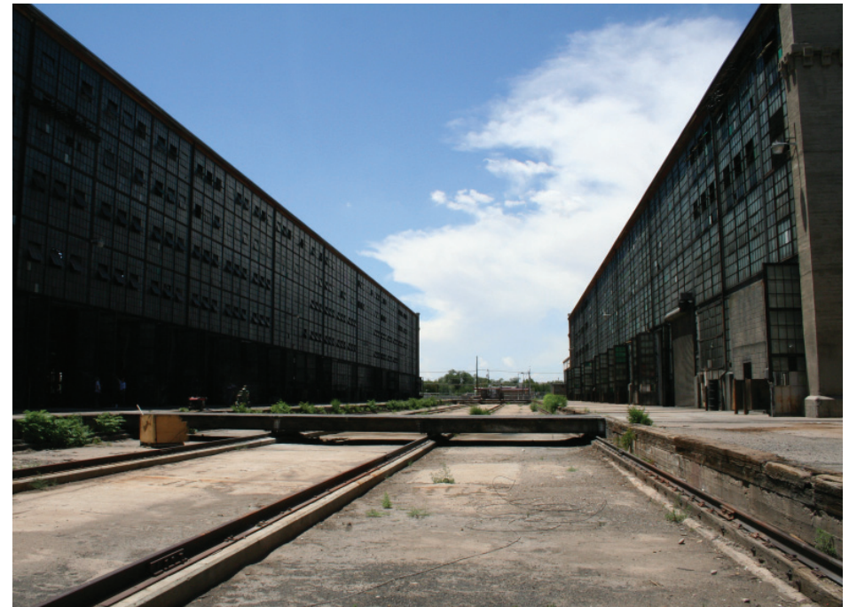
Transfer Table, View trough the East Side.
