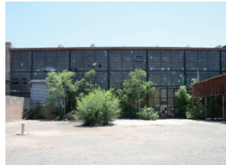
North elevation, Exterior courtyard in foreground.
