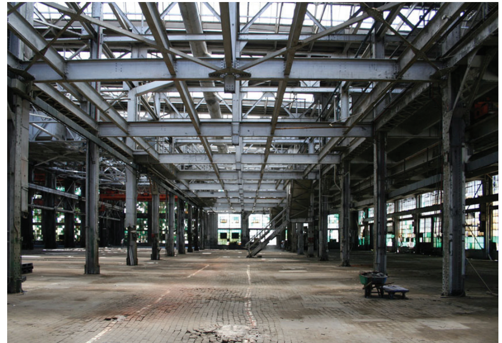
Machine Shop, Bay #2, Pyramidal skylights run between bays 2 and 3.
