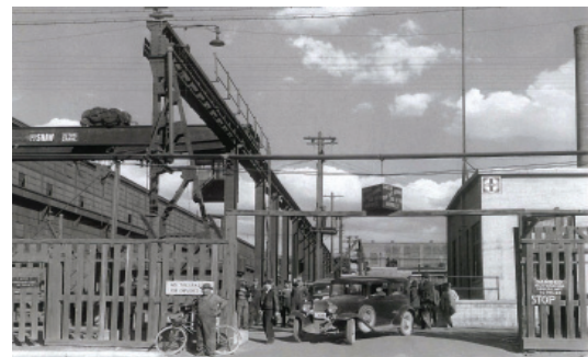
Historic Rail Yards Entrance
