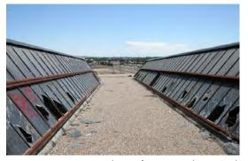
Built-up roofing, positive slope to South.
