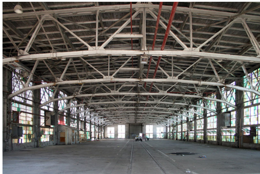
Blacksmith Shop, Steel Trusses, Wood Plank Ceiling, Glazed East and West elevations.
