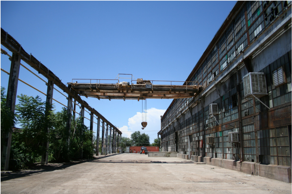
15 Ton Bridge Crane Connected to South Elevation of Machine Shop. Crane structure extends to 2nd Street.
