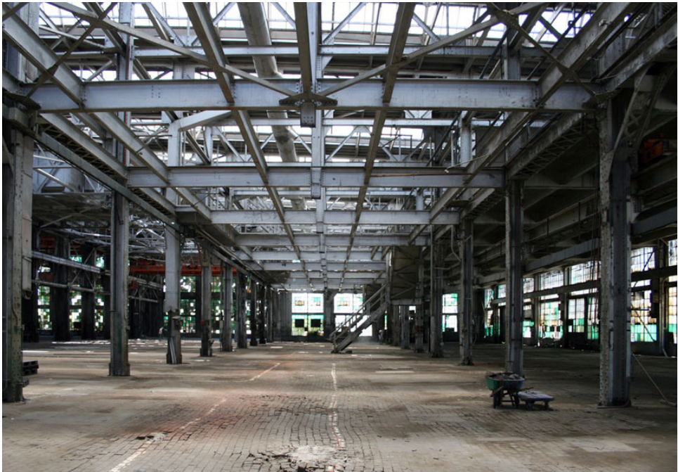
Machine Shop, Light Machinery Bay #2, Pyramidal skylights run between the Heavy and Light Machinery Bays bays 2 and 3.
