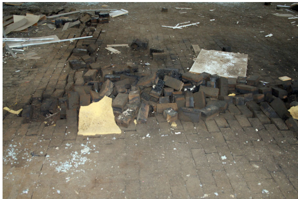
Damaged flooring, 3" thick creosoted end-grain wood blocks
