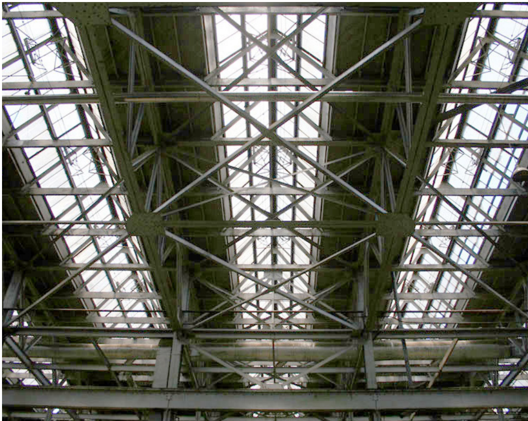
Machine Shop, Pyramidal skylights over the Heavy and Light Machinery Bays 2 and 3.
