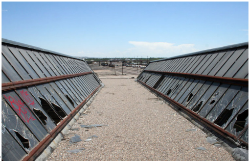
Built-up roofing, positive slope to South.
