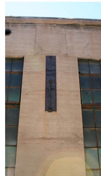
Steel plate seismic upgrades.
