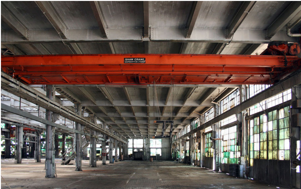
Machine Shop, Bench Bay #1 - Below board formed, cast in place, concrete mezzanine.
