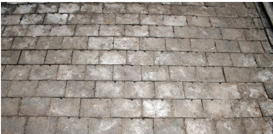
Flooring, 3" thick creosoted end-grain wood blocks.
