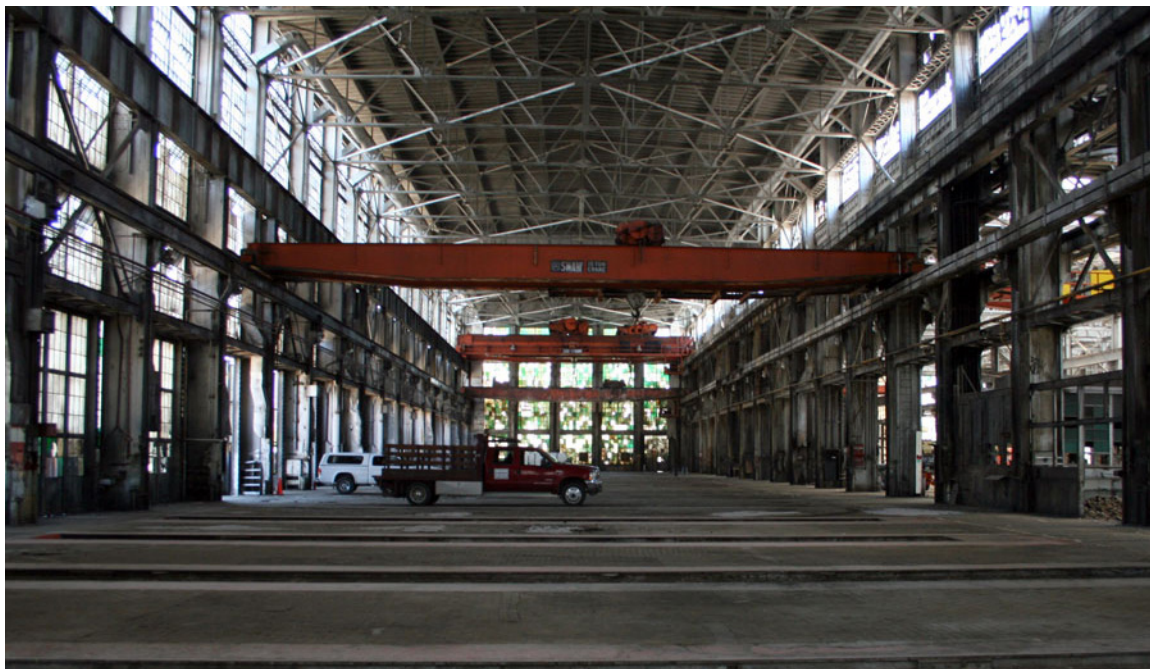
Machine Shop, Erecting Bay Bay #4, 57' clear height to underside of truss structure. Floor troughs can be seen across slab.
