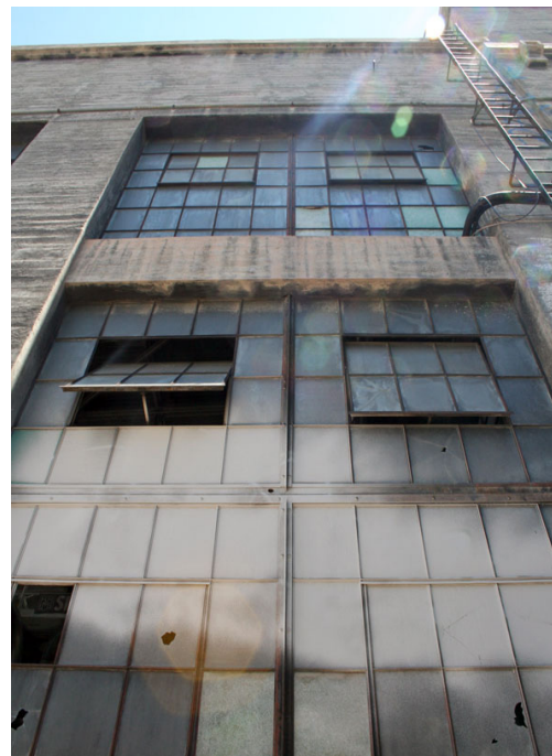
West elevation, Glazing inset to concrete frame.
