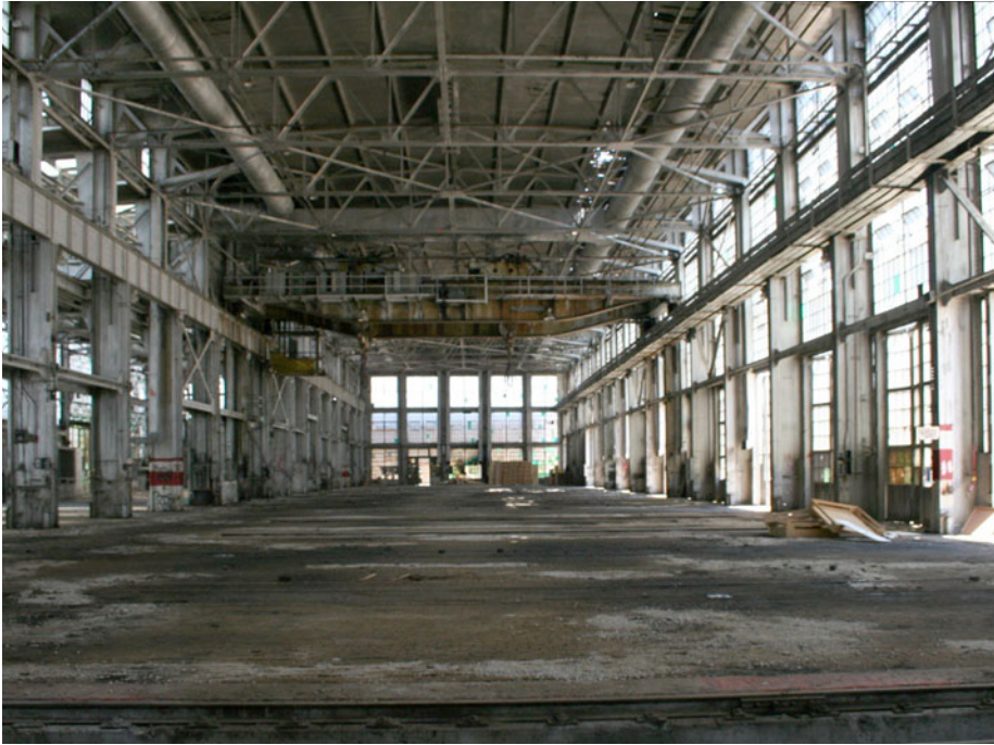
Boiler Shop, Erecting Bay Bay #1 , Fully Glazed southern elevation, Crane at rear. Floor troughs seen across
