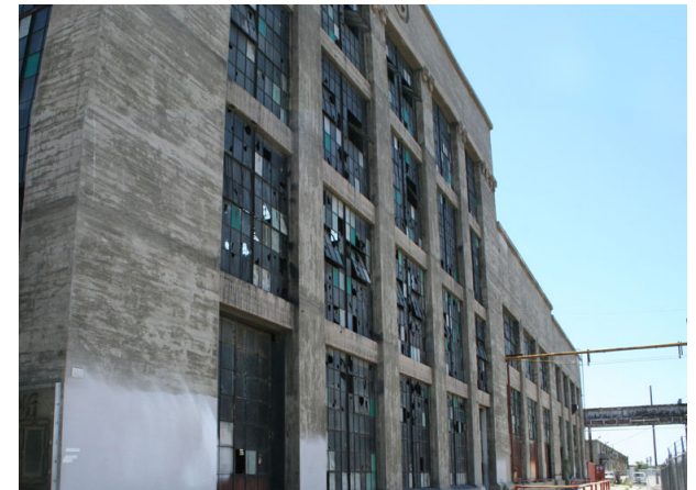
West Elevation, Cast in Place Concrete Frame.
