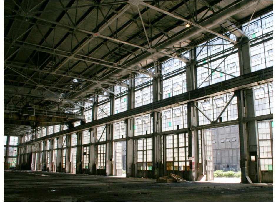
Boiler Shop, Erecting Bay Bay #1 , Fully Glazed southern elevation with 18' tall operable doors.
