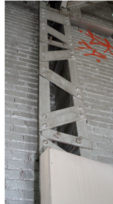
Steel 'trussed' column.
