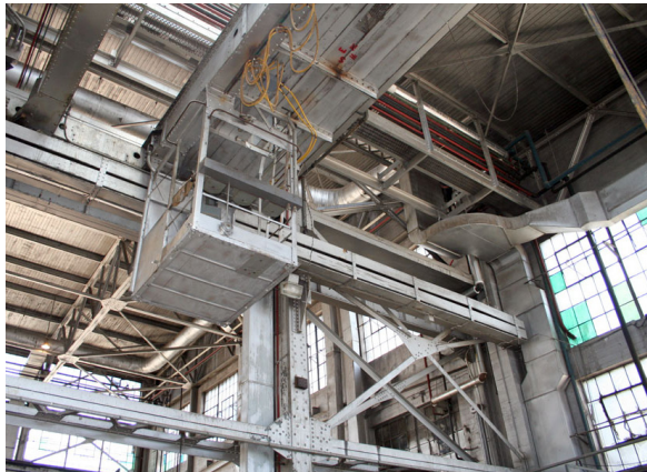
Crane operator workstation, Heavy Equipment Bay Bay #2.
