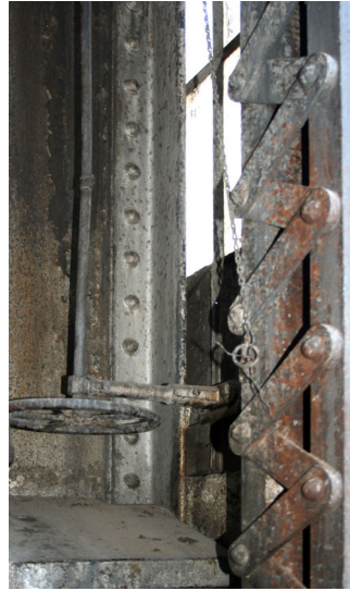
Crank mechanism for skylight operation.
