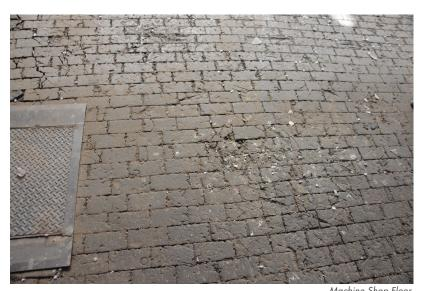
Machine Shop Floor, 3" thick Kreolite creosoted woods blocks sit on a 6" thick concrete floor to dampen sound
