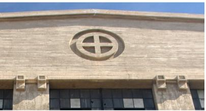
Cast-in-place concrete structure of Machine Shop with integral logo
