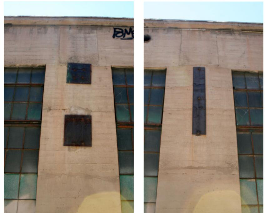
*Steel plate seismic upgrades.*
