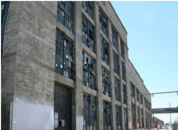
West Elevation, Cast in Place Concrete Frame.
