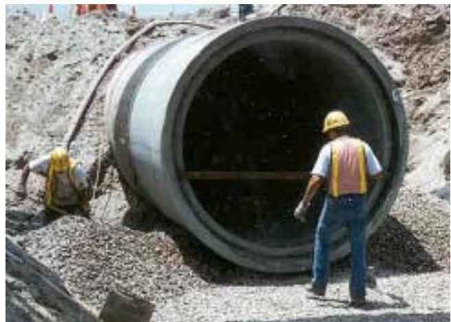
Sewer interceptor under construction
