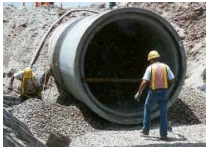
Sewer interceptor under construction
