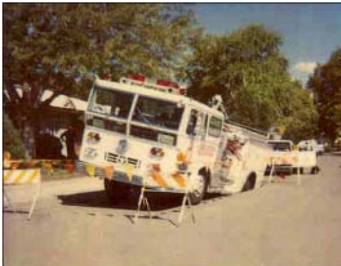
Street cave in at sewer rehab project.
