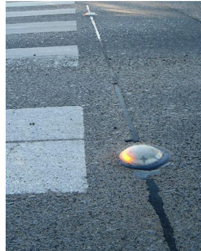
FIGURE 4-11 Example of Grade-Level Caution Lights
