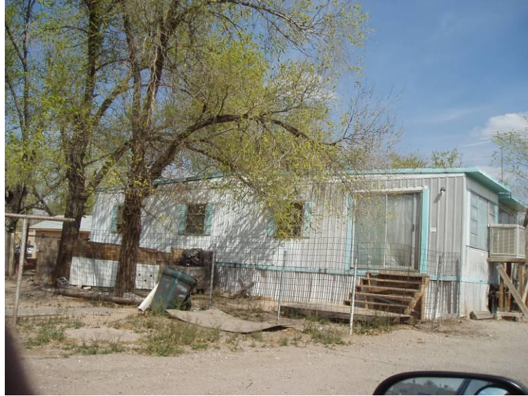
FIGURE 5-5 MOBILE HOMES IN POOR CONDITION
