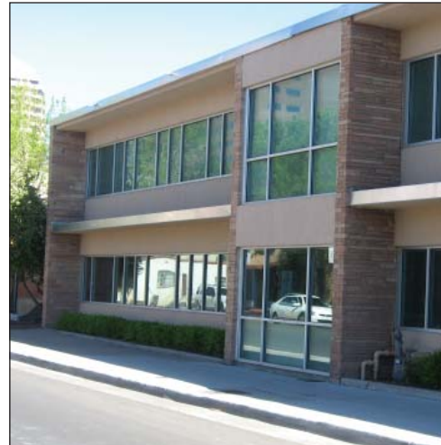
Office Building on Eighth St. - ground floor facade contains more than 50% of its surface in windows and 30% of the second story
