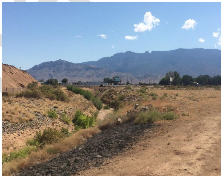
Figure 6 –Deteriorating drainage channel
