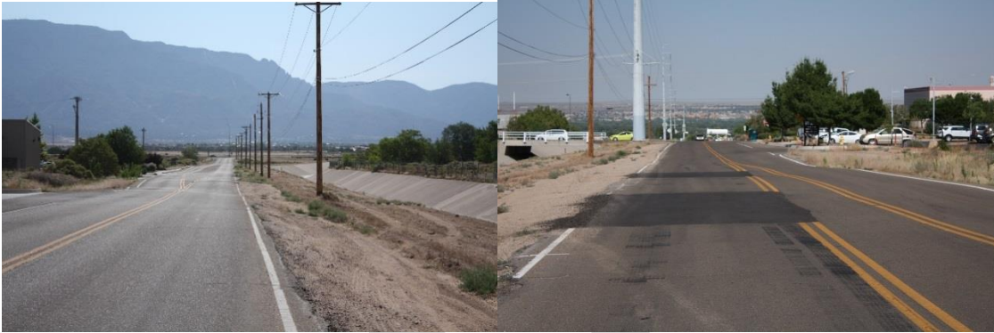
Figure 10 – Existing Conditions along San Diego Avenue
