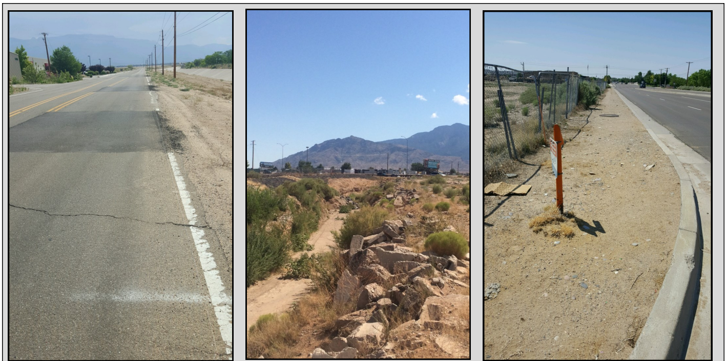
Figure 3. Infrastructure Deficiencies in the MR Area. From Left to Right: Expanding and Contracting Road Conditions, Deteriorating Drainage Channel, Lack of Sidewalks
