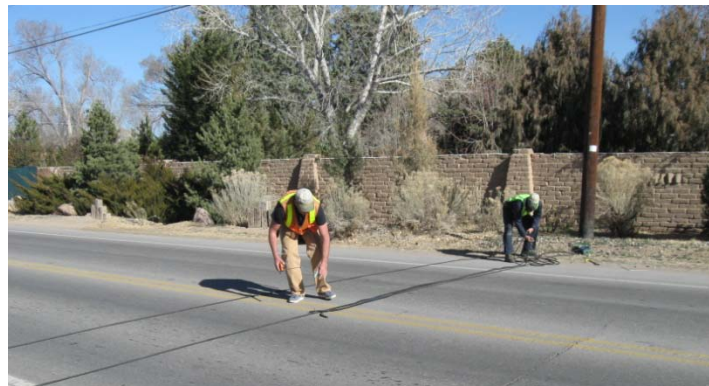
Pneumatic Tube being Place on Rio Grande Boulevard
