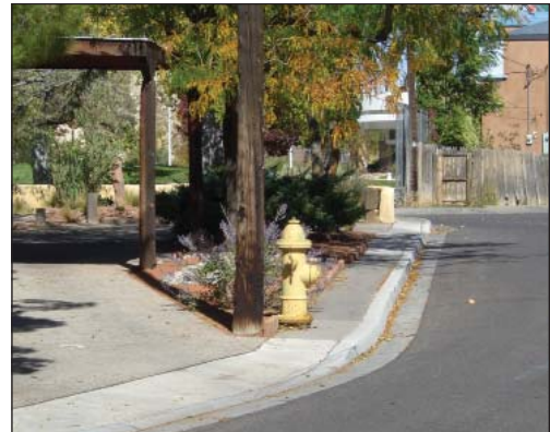
Fire hydrant obstructing very narrow sidewalk
