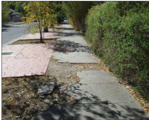
Deteriorated sidewalk
