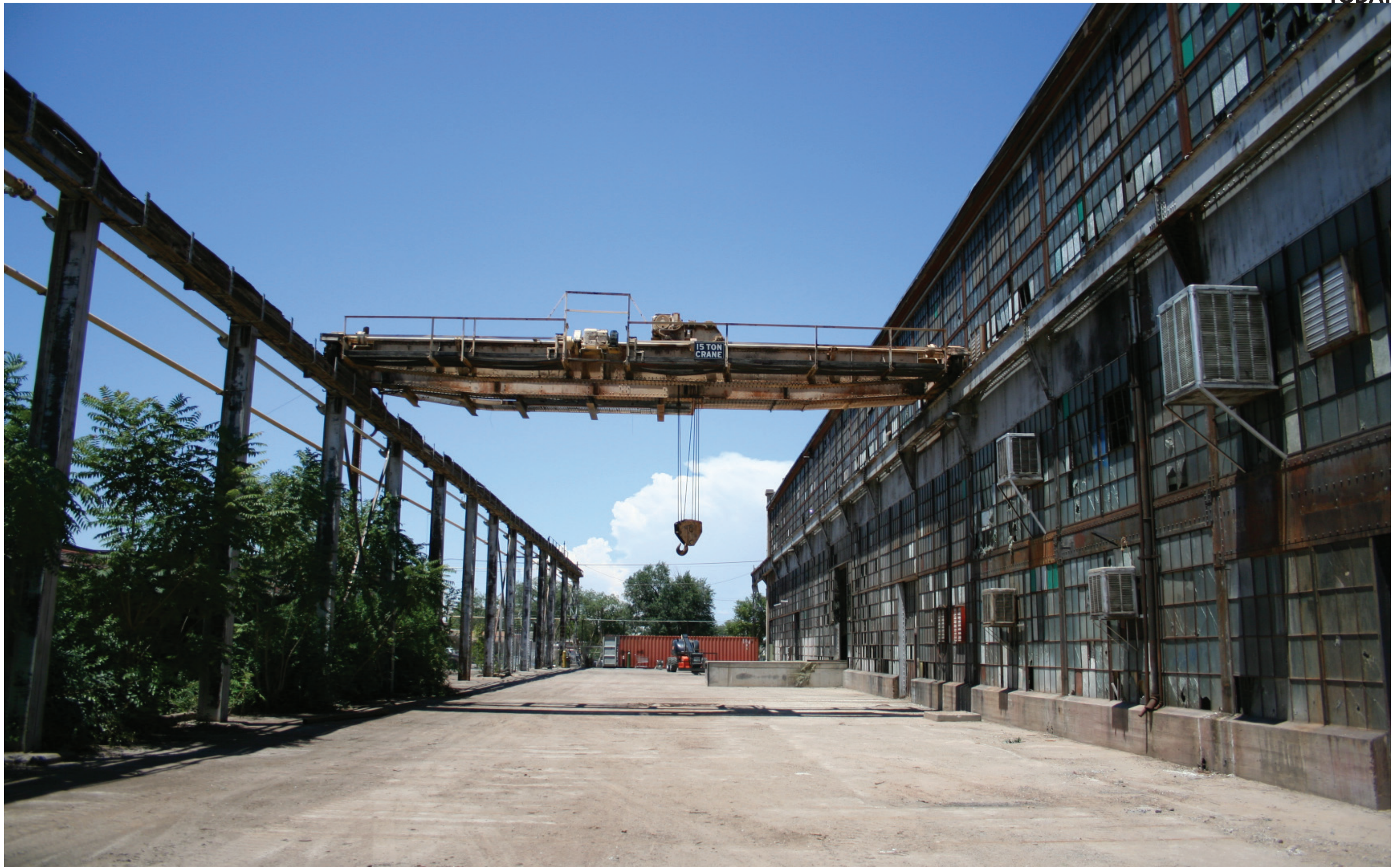
15 Ton Gantry Crane Connected to South Elevation of Machine Shop
