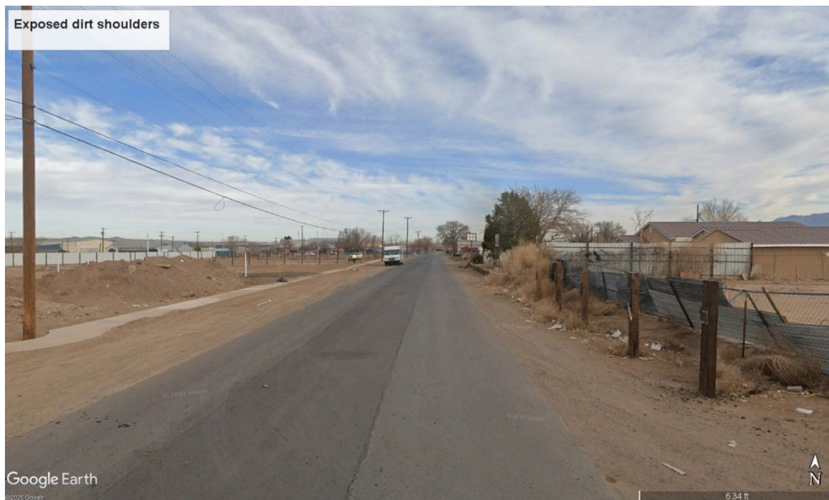
Figure 7: Street Near the 22V Monitor Showing Exposed Dirt
