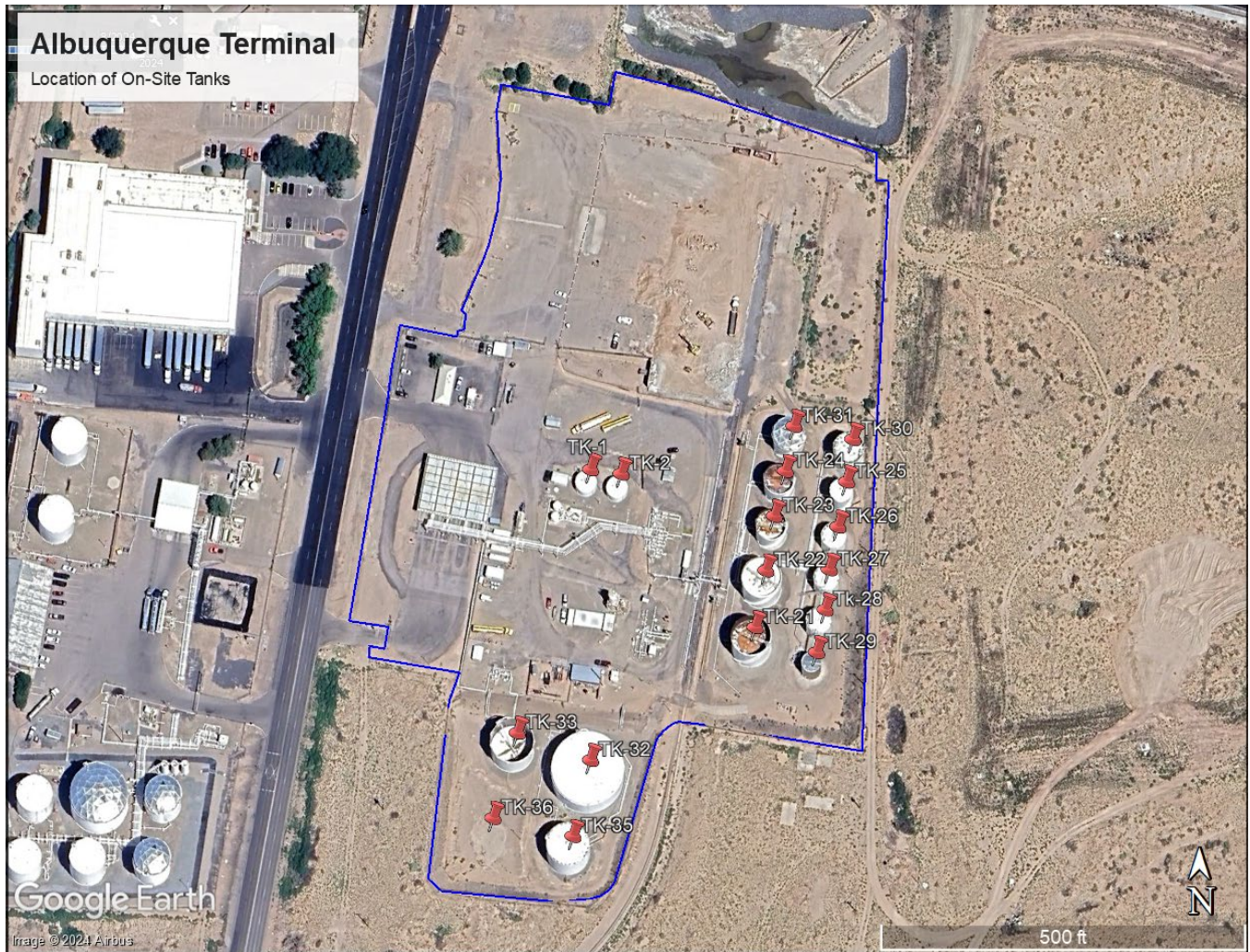
Figure 3. Location of On-Site Tanks
