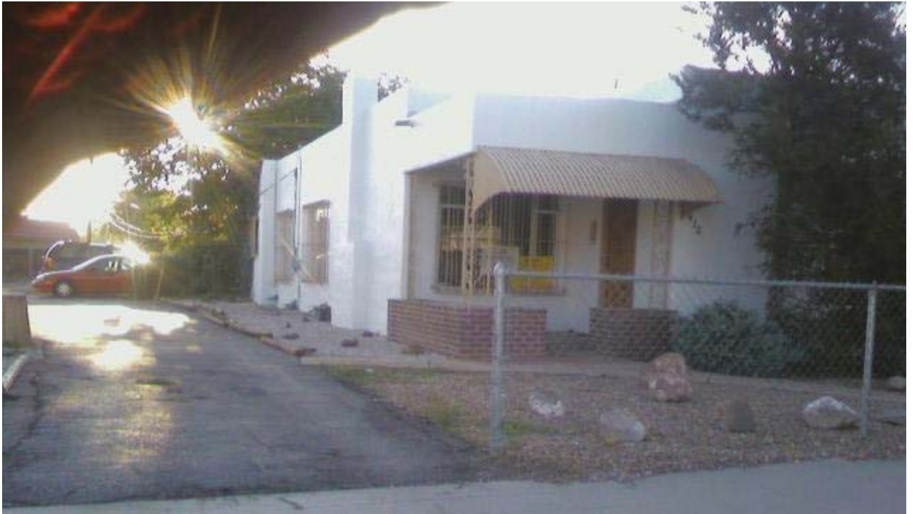
Above: View from Sixth Street, looking ESE.
