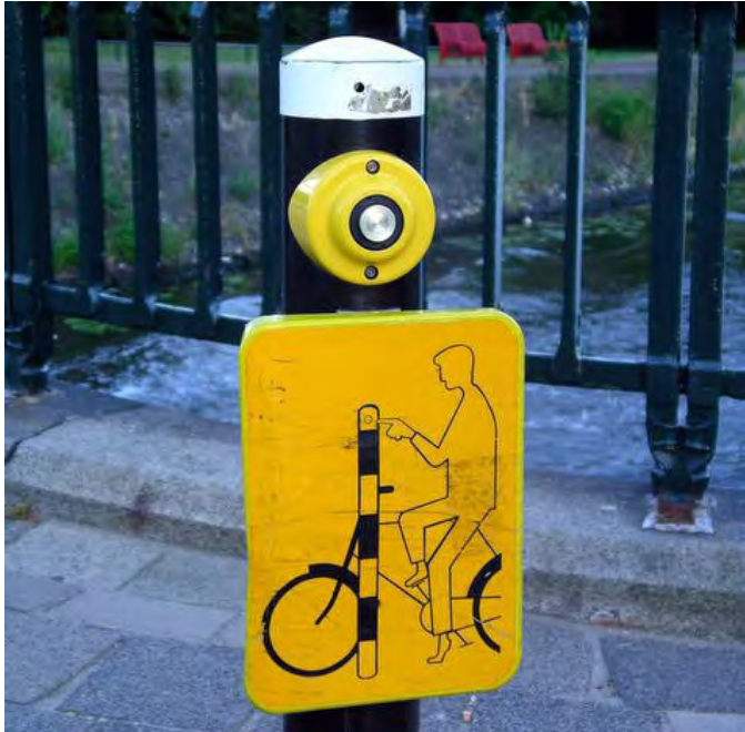
Example of curbside bike button.
