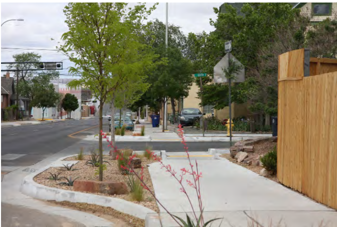
Bulbout improvement on Lead Avenue.
