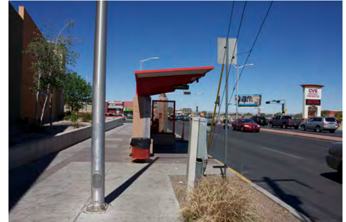
Transit shelter, light poles and other infrastructure outside of clear sidewalk area.
