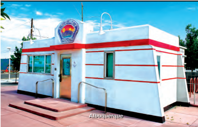
Triangle Substation, Nob Hill (1)
