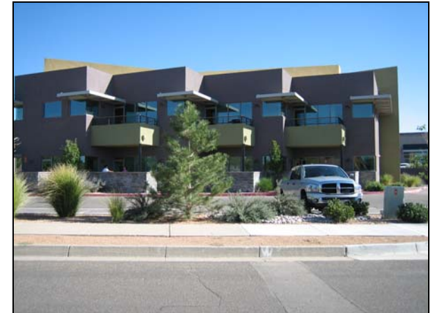
This building is divided into vertical segments, reducing the mass and providing interest from the street view.
