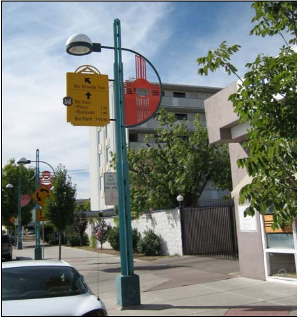
Site lighting should be design to facilitate safe and convenient circulation of motorists, bicyclists and pedestrians.
