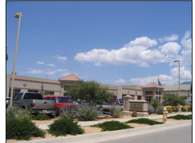
A landscape buffer should be provided between the street right-of-way and parking area
