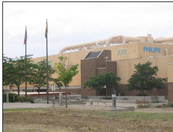
View of the former Philips plant, located near the intersection of San Mateo Boulevard and San Diego
