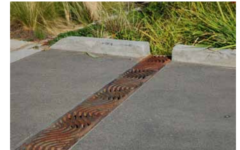
Decorative Grill and Curb Cut
