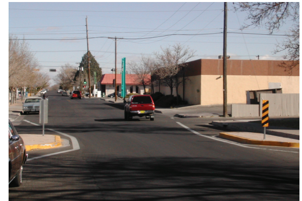
Traffic choker near Zia Elementary helps to slow traffic
