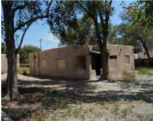
(12th and Major before demolition)
