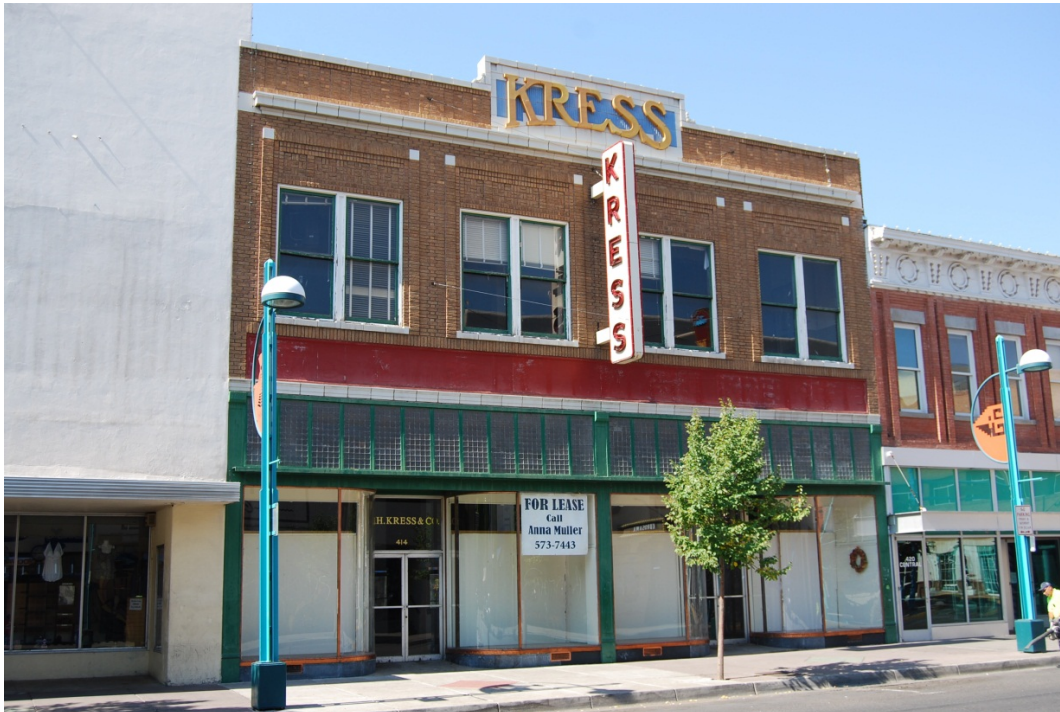
S.H. Kress Building, 414-416 Central SW
