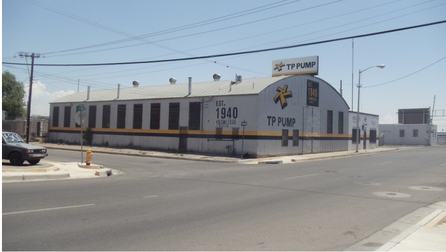
Former Eaton Metal Products building, 1824 2 nd St. NW (1939)
