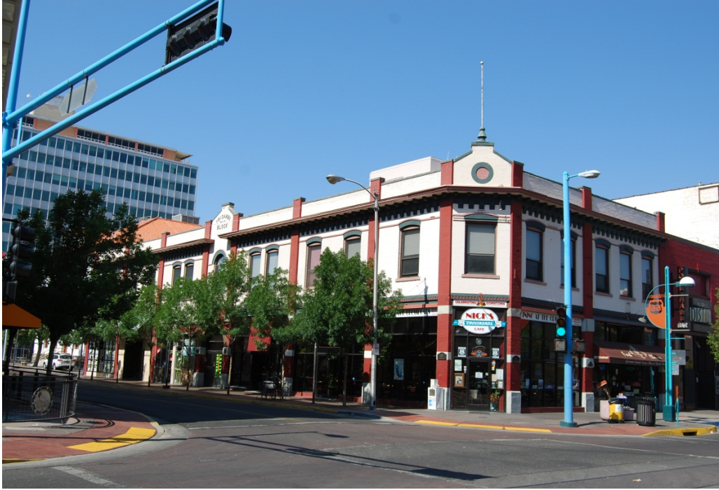
Yrisarri Building, 4 th and Central SW (ca. 1910)
