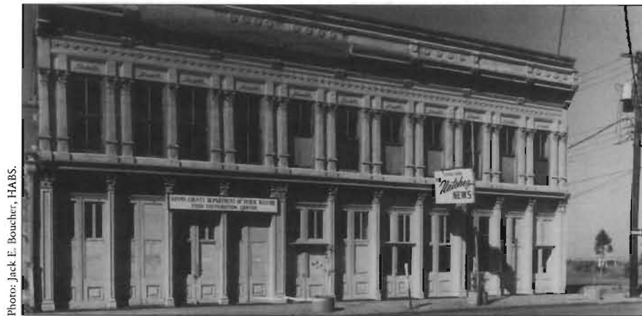
Deteriorated portions of the decorative pressed metal cornice have been inappropriately replaced with non-matching, plain metal sheets, adversely affecting the historic character of this building.
