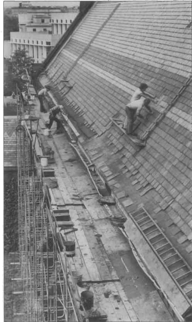
Workmen are in the process of removing deteriorated roofing slates and replacing them with new matching slates.
