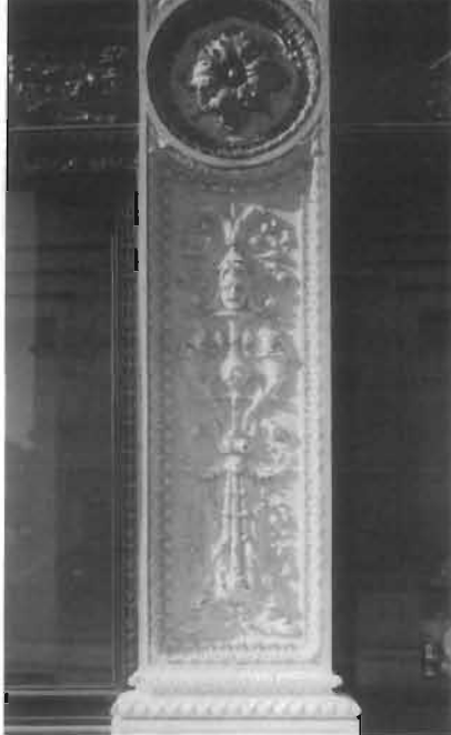
The decorative cast-iron storefront column was sandblasted in order to remove flaking paint and rust prior to repainting. Unlike soft metals such as copper and tin, which are damaged by abrasive cleaning, sandblasting is an appropriate method for cleaning cast iron, a very hard metal.
