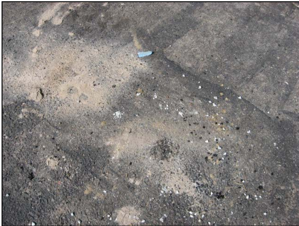
No. 4 – View of a typical asphalt patch using cold patch asphalt.
