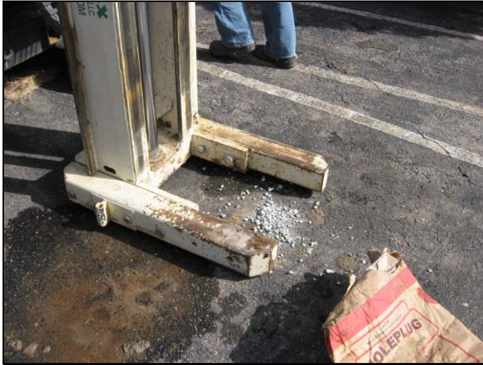
No. 3 – View of abandoning a soil boring with bentonite pellets.
