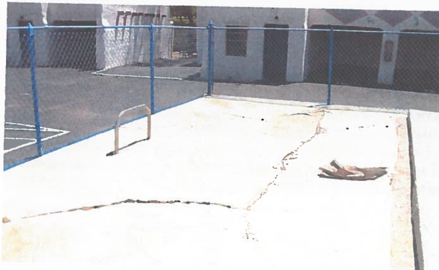
Figure 13 Cracked Concrete at Swimming Pool deck
