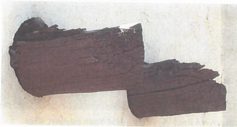
Figure 22 Dry Rot Viga Ends
