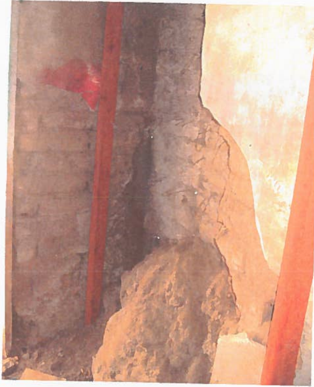
Figure 19 Collapsed Storage Shed Adobe Walls
