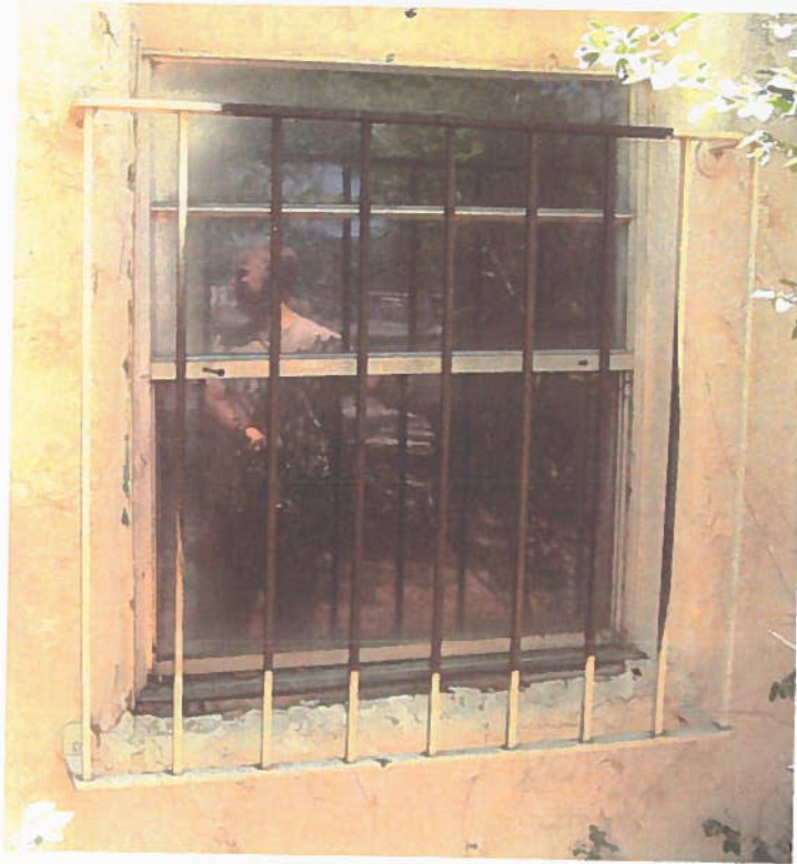
Figure 45 - Single Hung Window With Security Bars
