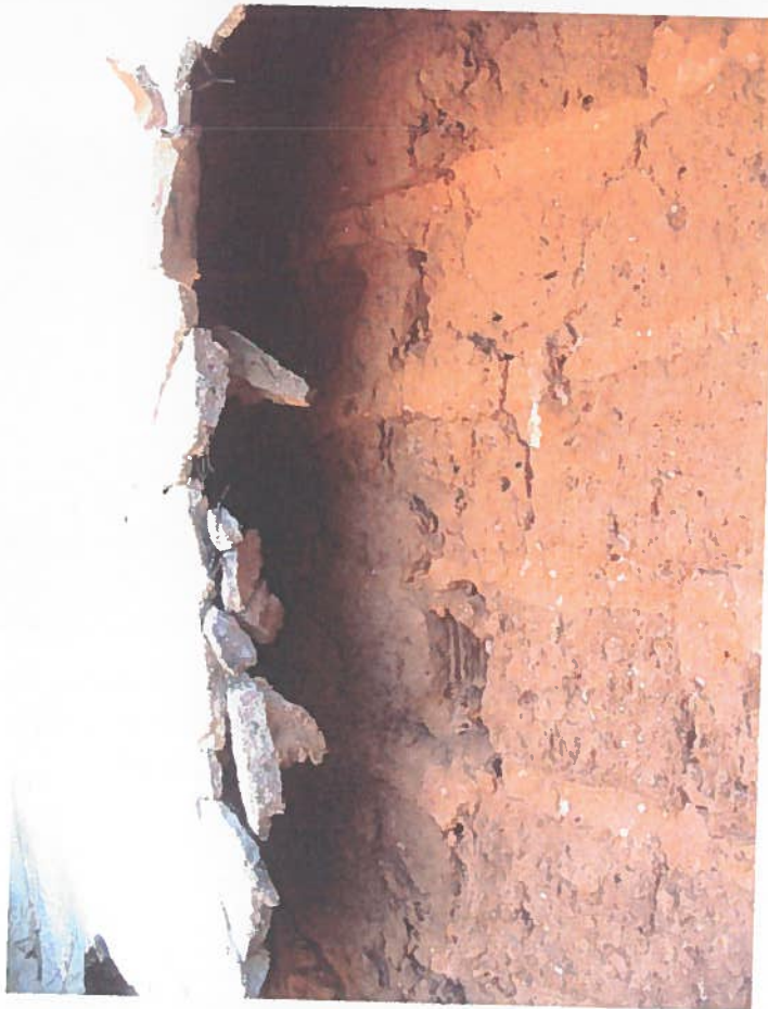
Figure 39 - Cement Stucco Separation from Adobe Wall
