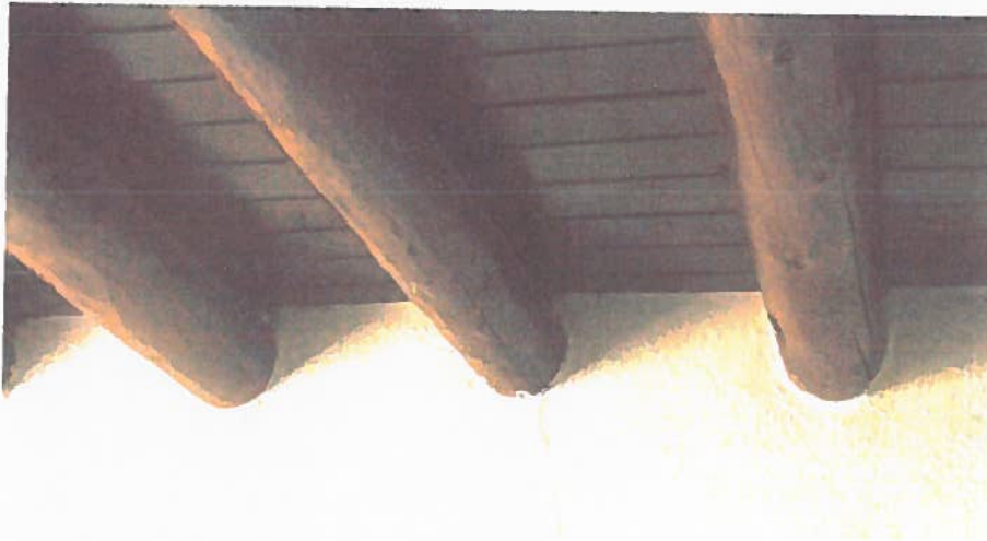
Figure 21 Typical Viga Layout
