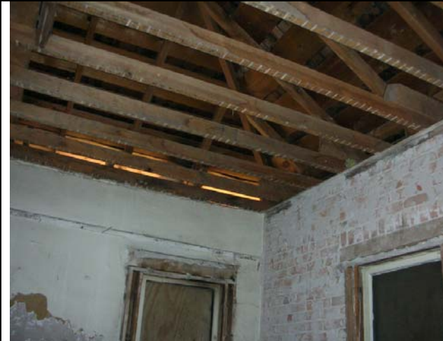
Interior at southeast
