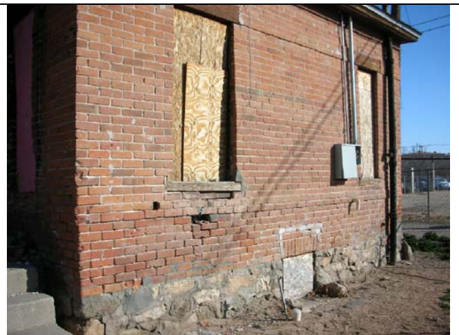
West façade, bowed horizontally and vertically
