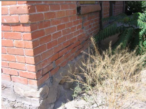
Typical stone foundation comprised of various stones with eroding mortar
