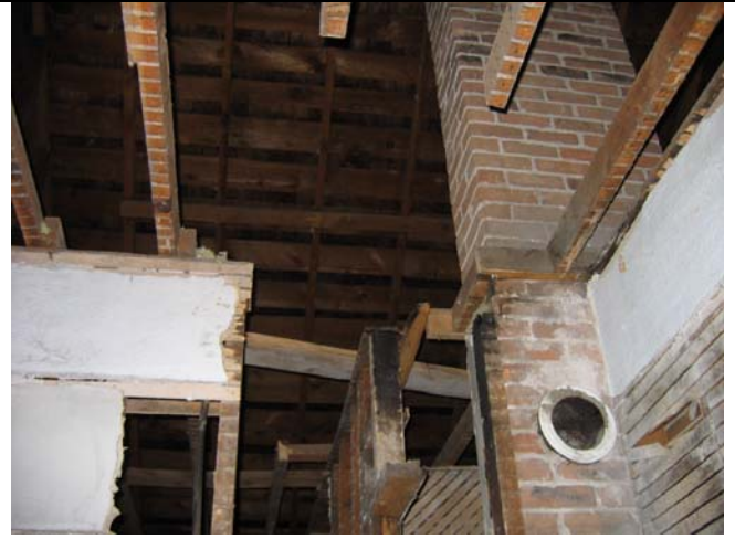
Interior brick flue, fire damaged bottom chords removed
