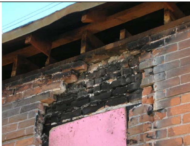
Window header fire damage at northwest facade
