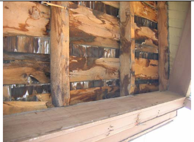
Front porch roof deck
