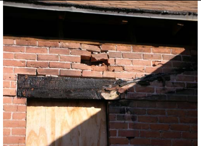
Fire damage at northwest porch
