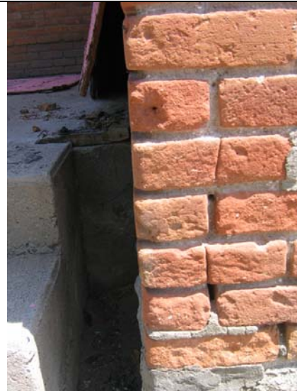
Brick and mortar erosion
