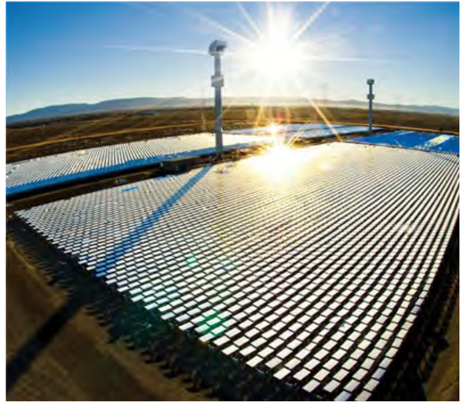
Concentrating Solar Tower Facility
