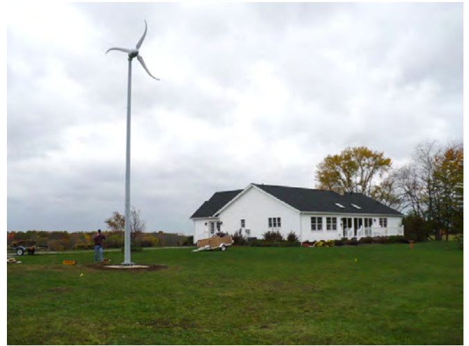
Wind Generation Installation
