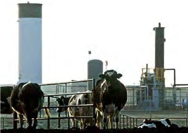
Biogas (Commercial Dairy Byproduct) Facility
