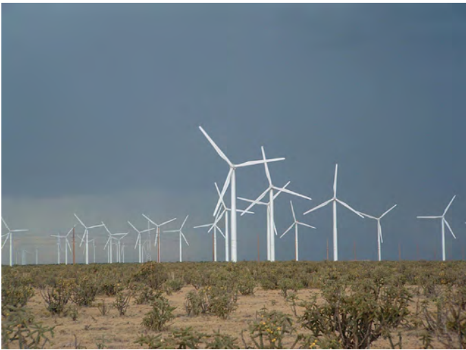
Wind Generation Facility
