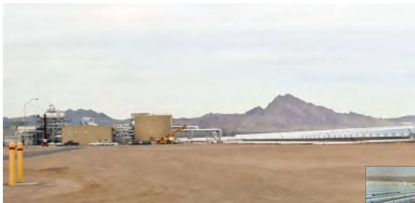
Concentrating Solar Linear Concentrating System Array Powering a Traditional Steam Turbine Generating Station
