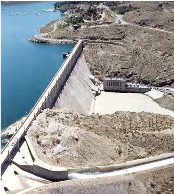
Hydroelectric Generating Station
