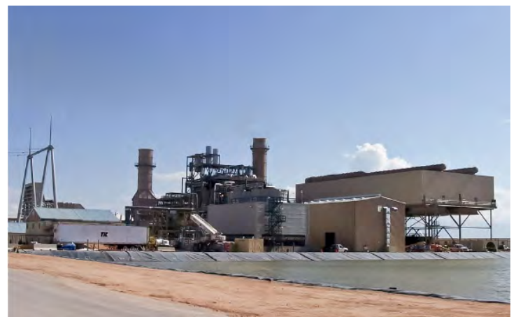
Combined-Cycle Natural Gas Generating Station
