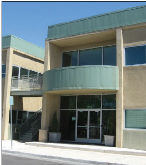
Office Building on Tijeras Ave. - entry is the predominant feature and faces sidewalk
