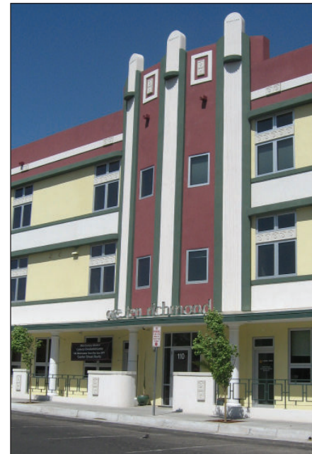
Vertical Mixed Use with office/retail on ground floor and apartments above. Top: Brick Light District on Harvard St. Bottom: 110 Richmond
