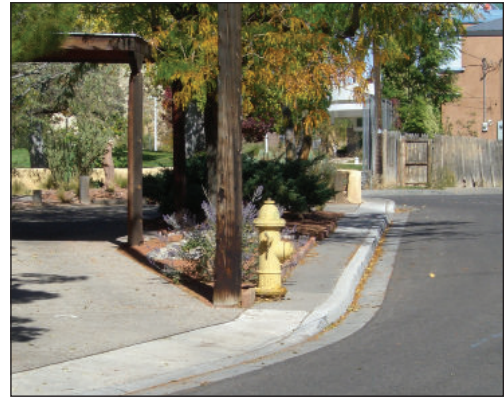
Fire hydrant obstructing very narrow sidewalk
