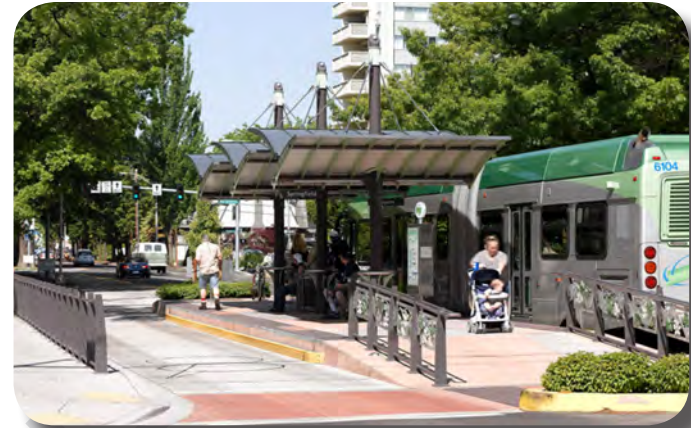
Example of a median BRT station with a shelter, seating and ADA accessibility in Eugene, Oregon
