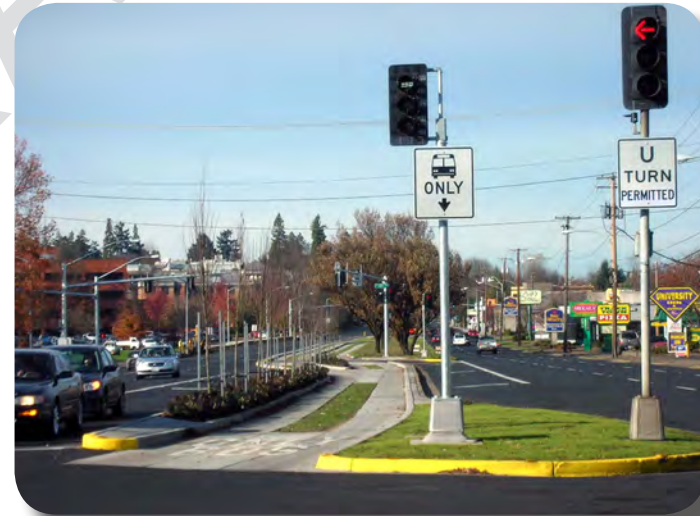
Example of a median-running BRT lane at a signalized intersection in Eugene, Oregon
