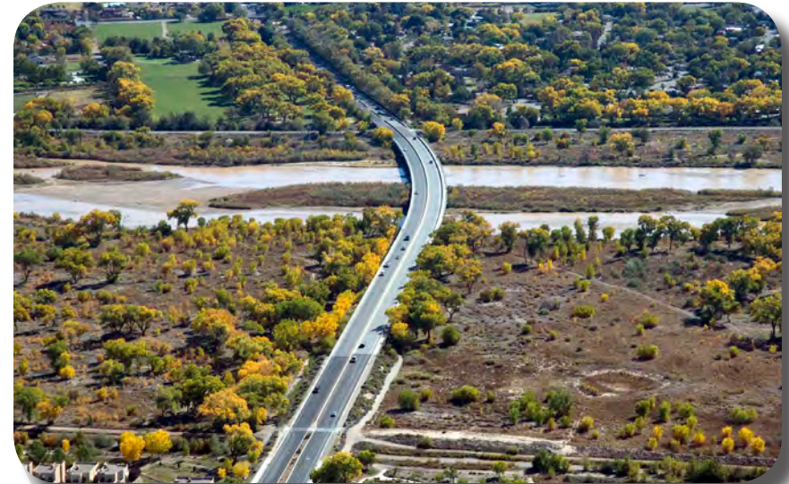
River-crossing capacity is key to providing regional mobility to and from the West Side.
