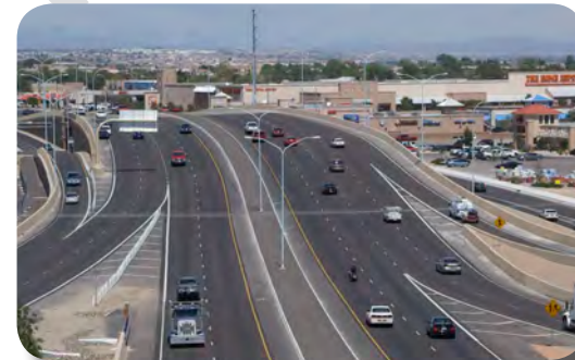
View of the I-40/Coors Boulevard interchange ramps south of the Ouray underpass
