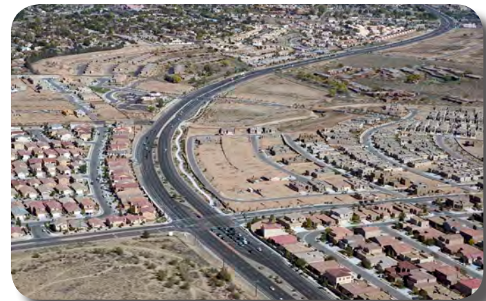
Aerial view of Coors Boulevard at Western Trail/Namaste Road
