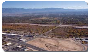
Aerial view of the Rio Grande Bosque at the Montaño Road river crossing.
