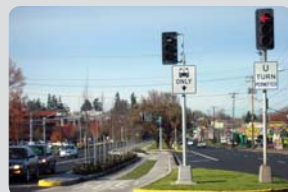
Example of a median-running BRT lane at a signalized intersection in Eugene, Oregon
