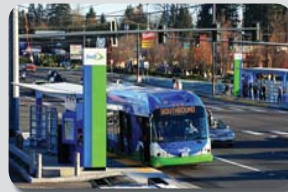
Example of a curbside-running BRT lane at a station in Everett, Washington
