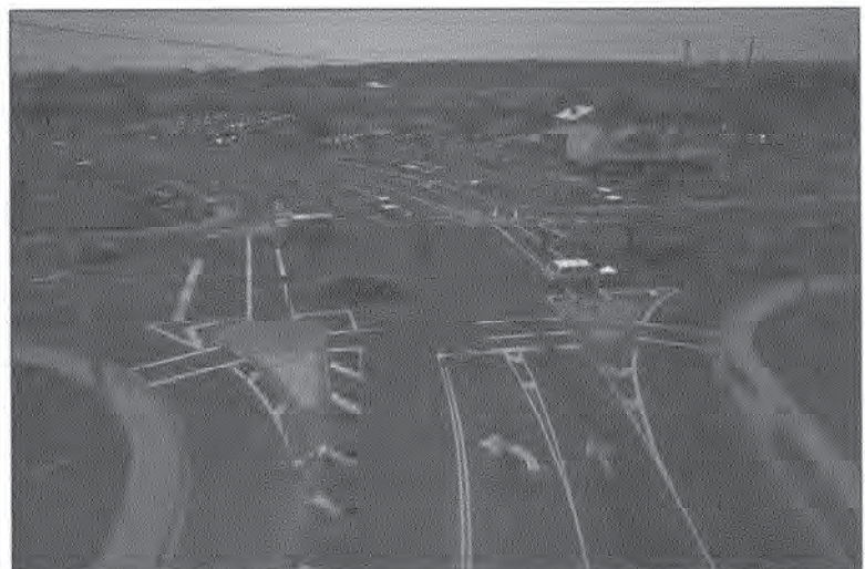
FIGURE 1-9. Properly designed right-turn slip lanes with pedestrian refuge islands can enhance crossings for pedestrians.
