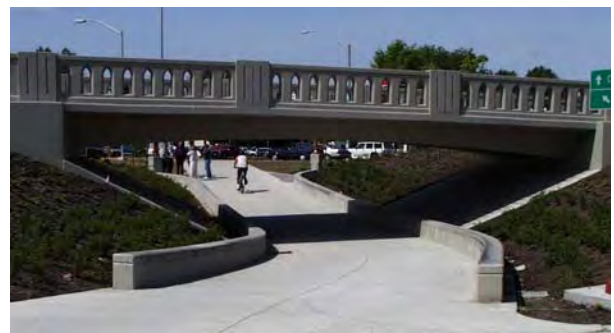
Figure 2-11 Grade-Separated Undercrossing (Example)
