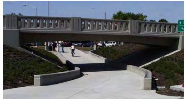
Figure 2-11 Grade-Separated Undercrossing (Example)
