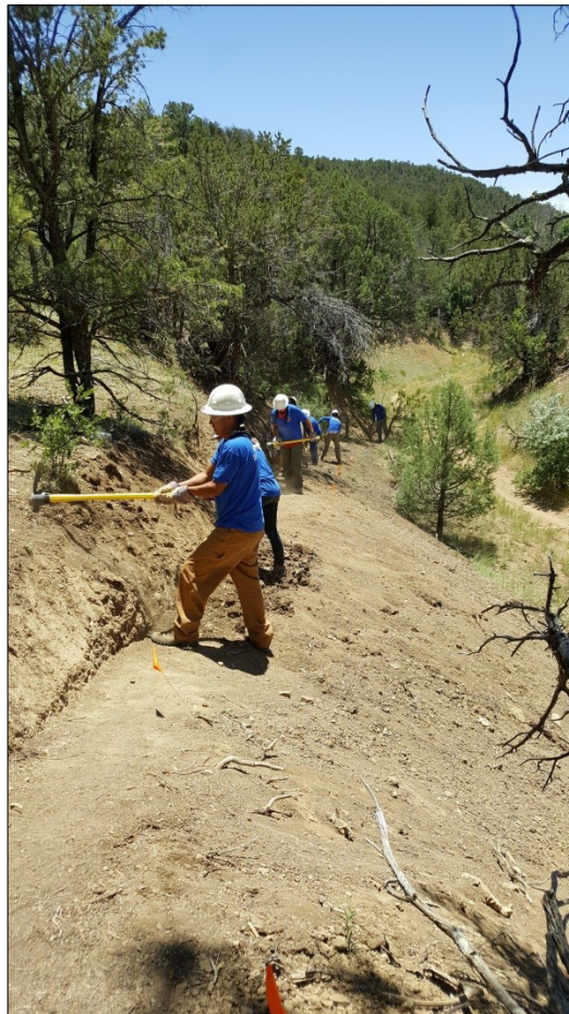
Rocky Mountain Youth Corps crew building the new trail at Milne Open Space Photo by Jim Sattler
