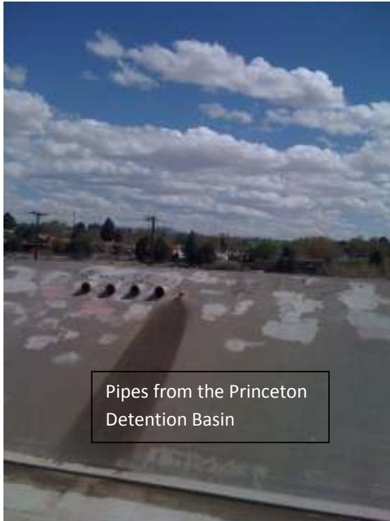
flowing directly into the valley area immediately to the west. Impounded water is collected at various locations and pumped into the NDC. Five pipes protruding from the south wall of the NDC mark the Princeton Detention Basin, maintained by the City, which is barely visible beyond the south wall. Water accumulating in the Basin is pumped into the NDC.
