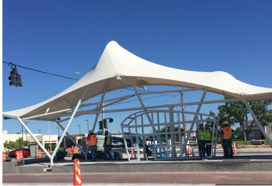
The canopy at Central and Coors is the first one to be installed along the ART route. FabriTec Structures of Dallas, Texas is handling the canopy installations, utilizing marine-grade steel for the framework. The canopies themselves are made of polytetrafluoroethylene, a Teflon®-coated, woven fiberglass membrane that is extremely durable and weather resistant. The canopies are designed to stand up to scorching desert heat, and are fire-resistant, as well.
