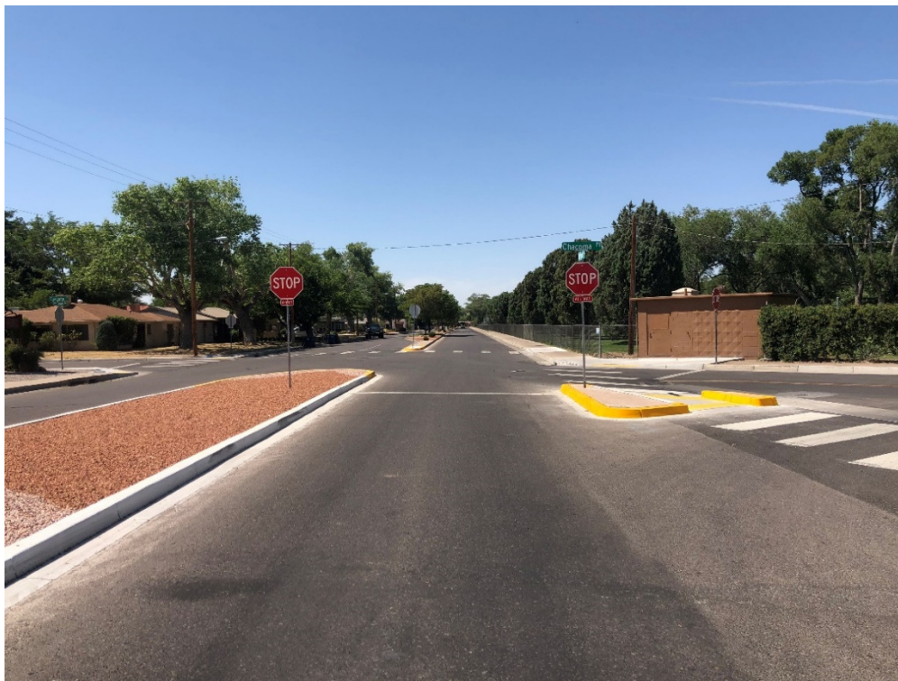
Figure 3: San Pasquale Avenue looking south
