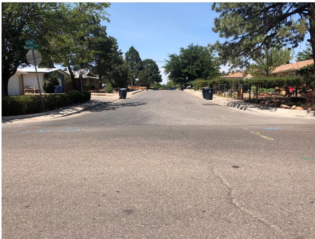
Figure 4: San Pablo looking north
