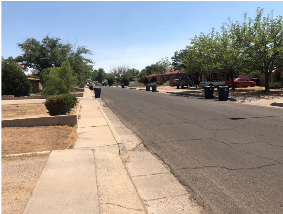
Figure 4: Quincy Street looking south
