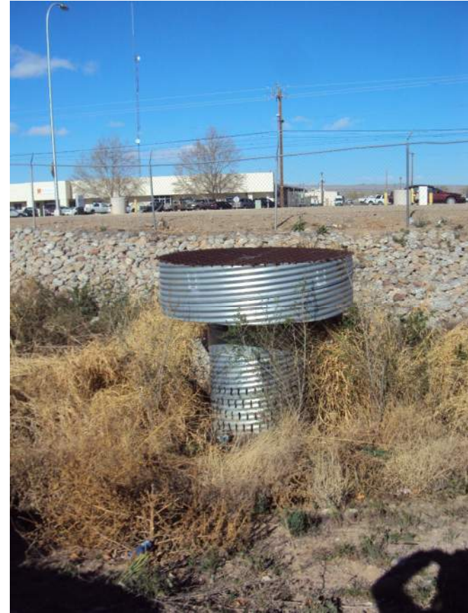
IMG_336: Overflow structure at the northwest stormwater detention basin
