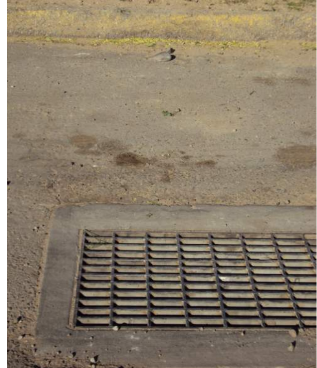
IMG_285: Storm drain on western portion of the site
