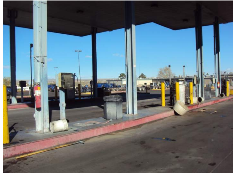
IMG_307: Fueling area
