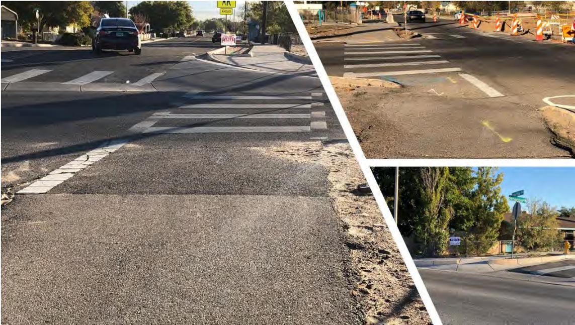
**Photo 2- Existing Non-ADA Compliant Curb Ramps**
