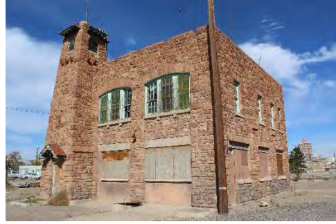
Figure 2 Exterior of Fire Station
