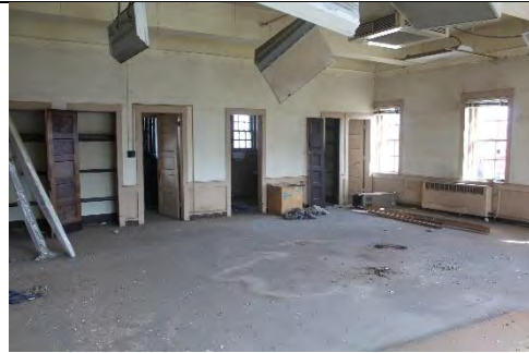
Figure 4 Interior of Fire Station
