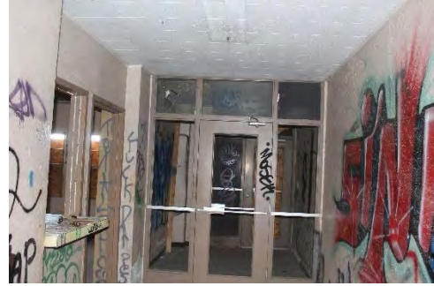
Figure 2 Entrance to Cab Paint Shop
