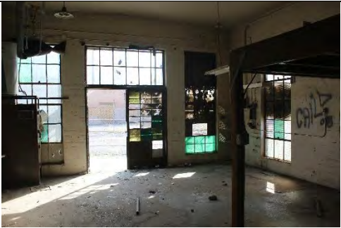
Figure 3 Interior of Waste & Paint Rooms
