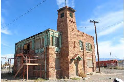
Figure 1 Exterior of Fire Station
