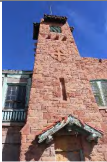
Figure 3 Exterior of Fire Station
