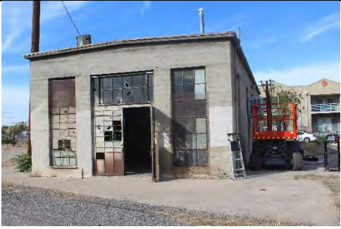
Figure 1 Exterior of Waste & Paint Rooms
