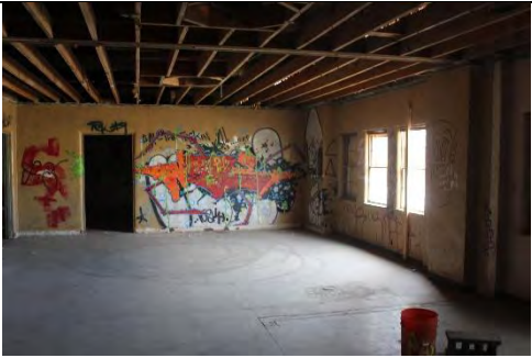
Figure 3 Elevated view of Interior of Tender Repair
