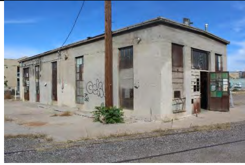
Figure 2 Exterior of Waste & Paint Rooms
